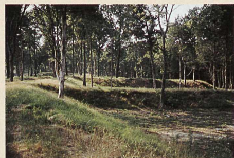
Curtain Wall No. 2 and traverse, Fortress Rosecrans
