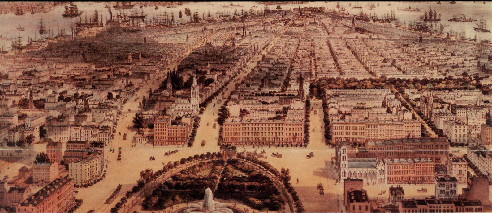
The scene above shows the neighborhood in which TR grew up, his home is off the picture in the center foreground. His grandfather Cornelius lived in the house just above the large tree at the end of the park. —J. Clarence Davies Collection, Museum of the City of New York
