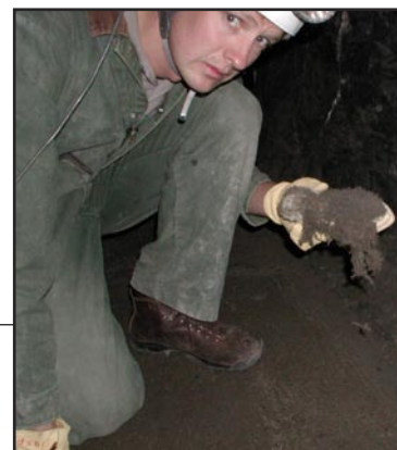
Lint and hair being removed from tunnel
