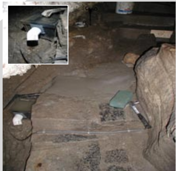
The finished drainage restoration at Salt and Pepper Shakers
