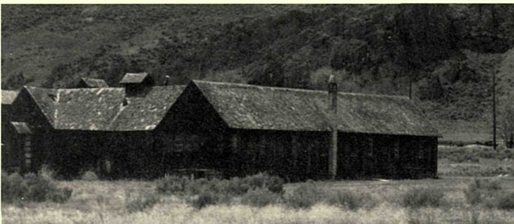
Camp Tulelake barrack prior to the start of restoration work
