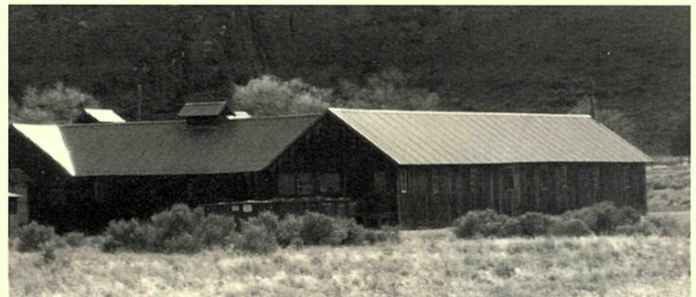
Camp Tulelake barrack during restoration work
