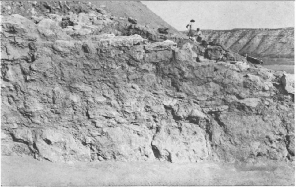
Detail of masonry.
