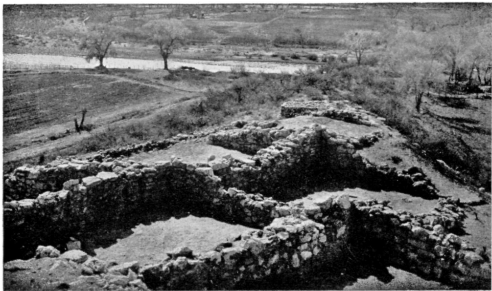
South end of Tuzigoot after excavation.
