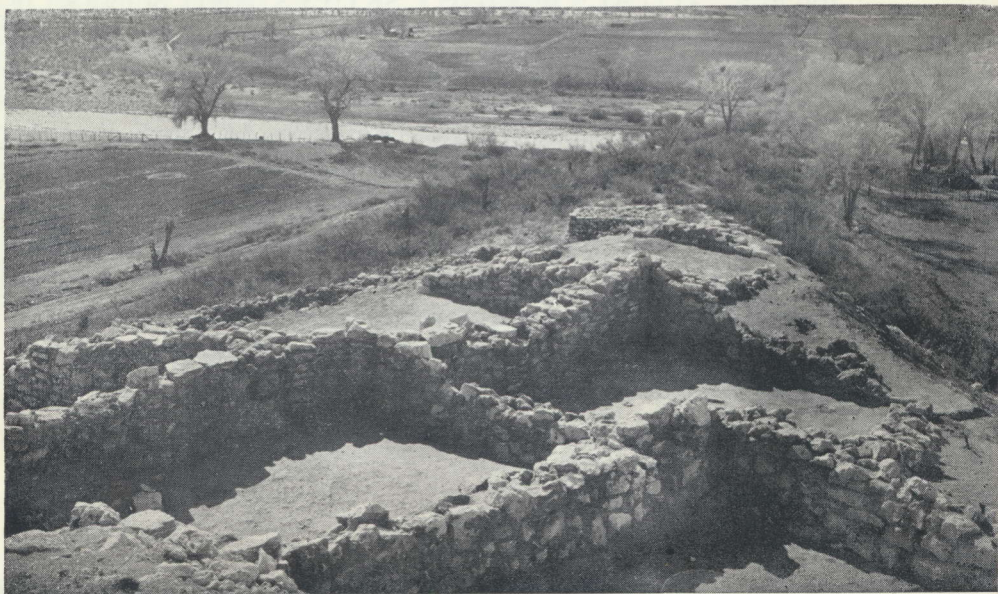
South end of Tuzigoot after excavation.
