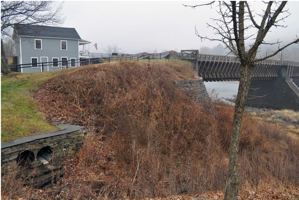
Figure 27. View looking southwest at the New York side of the former aqueduct and the rebuilt curved wing wall on the north side of the abutment. At image left is the culvert outlet that originates on Route 97. (OCLP 2014, DSC_0660)
