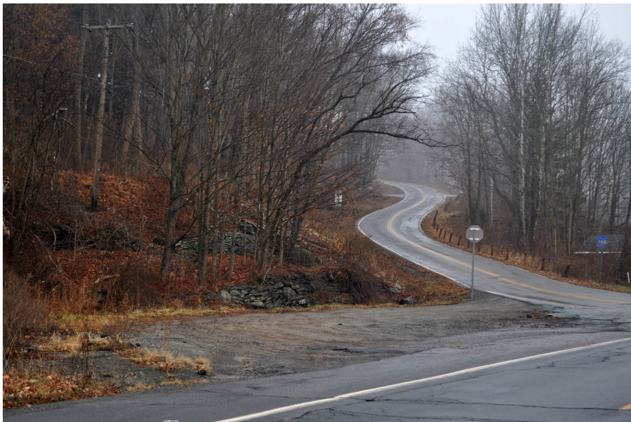
Turning basin and towpath walls at the intersection of Route 79 and Old Minisink Road.
