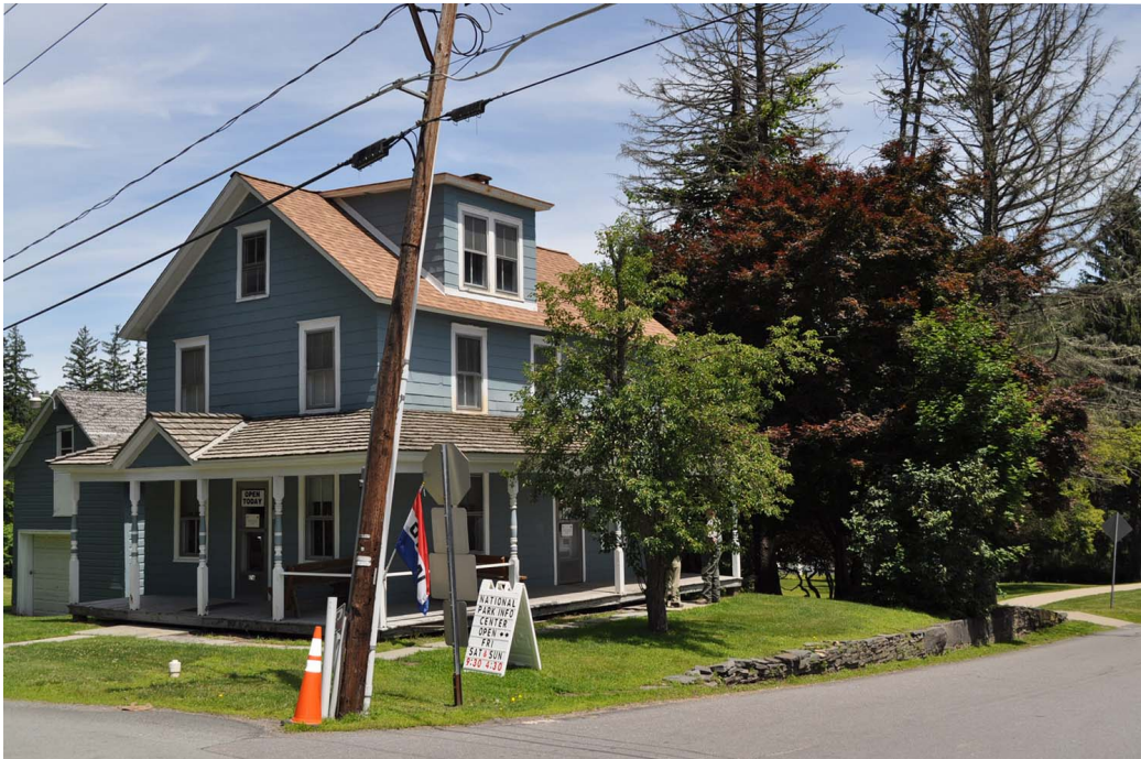
Figure 36. View looking northeast at the Margold house and garage, from Scenic Drive. The stone wall on the south edge of the yard wraps around to the east side of the yard. (OCLP 2014, DSC_0431)
