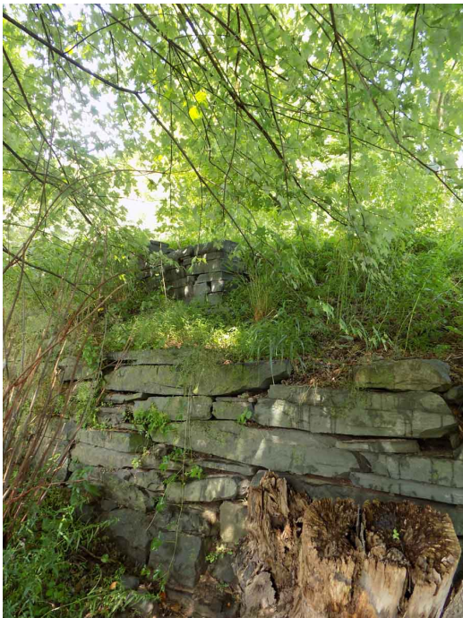
Figure 34. View looking northwest at an extant stone wall associated with the old towpath, upstream from Roebling's Delaware Aqueduct. The wall behind it (background) is contemporary and supports a maintenance access road. (UPDE 2016)
