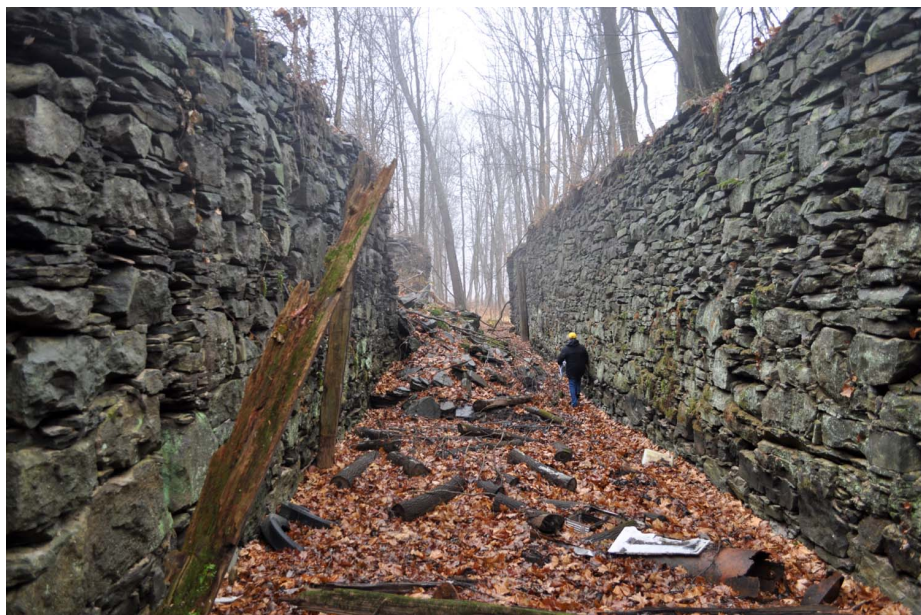
Interior view of Lock 71.
