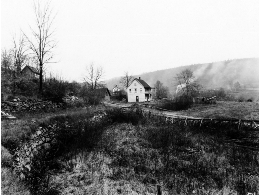
Figure 16. View looking south, 1923, at Minisink Ford Road passing through the former turning basin on the New York side. Walls associated with the turning basin and towpath are at image left. (Minisink Valley Historical Society, P-82-8-5)
