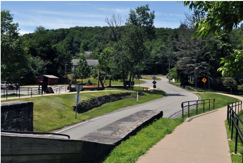
Figure 30. View looking west-southwest at the new canal prism wall and towpath on the south side of Delaware Drive. The Pennsylvania side parking lot, restroom, and bridge sculpture are visible in the background at image left. (OCLP 2014, DSC_0421)
