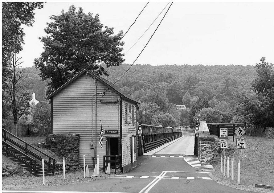
Figure 22. View looking west at the tollhouse and former aqueduct after it reopened to vehicular traffic, c.1988, before the towpaths were reconstructed (1994). (HAER PA-1, 1988, 123818pv)
