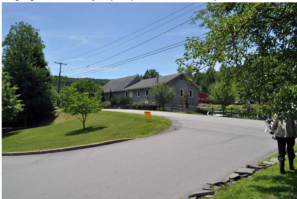
Figure 38. View looking southwest at the maintenance building. (OCLP 2013, DSC_0447)
