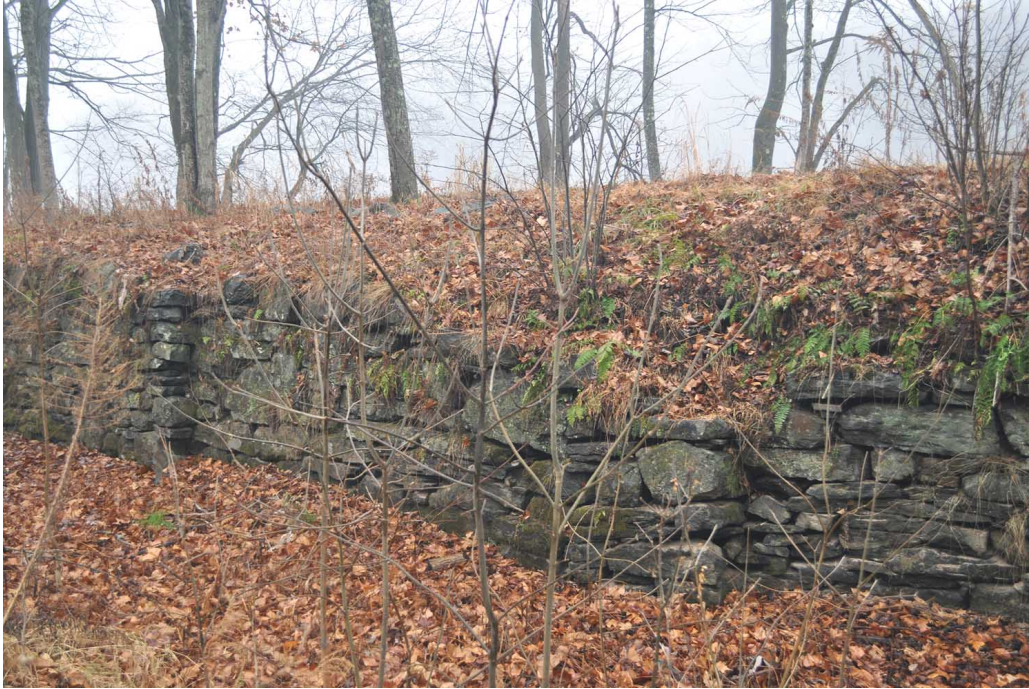
Figure 33. Close up view of a canal wall. Located just south of the current diversion dam, it likely served both the old and new canal. Note the recessed portions of the wall. (OCLP 2013, DSC_0572)
