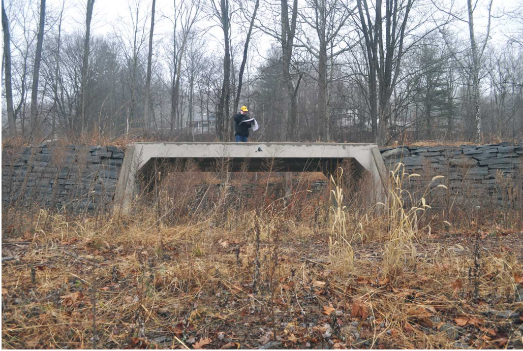
Figure 39. View looking east at the concrete box culvert at the breach in the old canal towpath. (OCLP 2013, DSC_0534)
