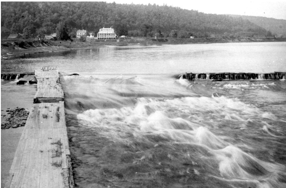
Figure 12. View looking north at slackwater dam and icebreaker at the western-most aqueduct pier, 1852-98. Note the two people next to the dam at image center and the Delaware House Hotel in background. (Minisink Valley Historical Society, P-98-8-18)
