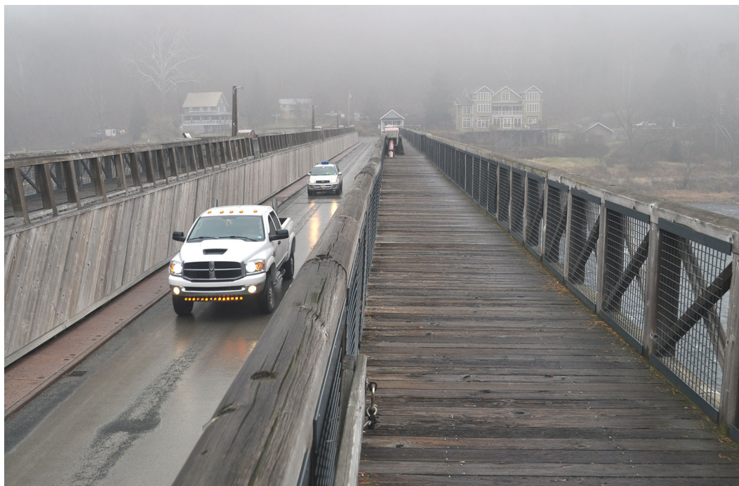
Figure 40. View looking east, from the towpath on the downstream side of Roebling's Delaware Aqueduct. (OCLP 2013, DSC_0288)
