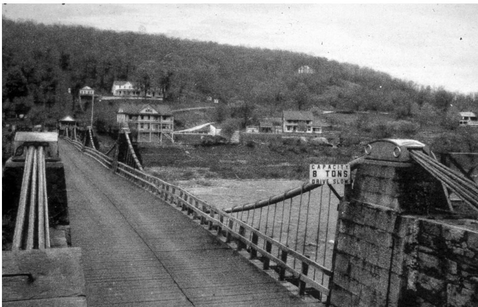
Figure 19. View looking east-southeast at the redesigned deck, c.1932. (Park Image File, Delaware & Hudson Canal, Historic Roebling Bridge, Scan 140)
