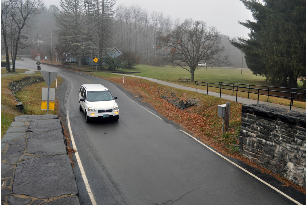
Figure 29. View looking west-northwest at two remnant stone walls associated with the new canal prism, on the Pennsylvania side of Roebling's Delaware Aqueduct. (OCLP 2013, DSC_0298)
