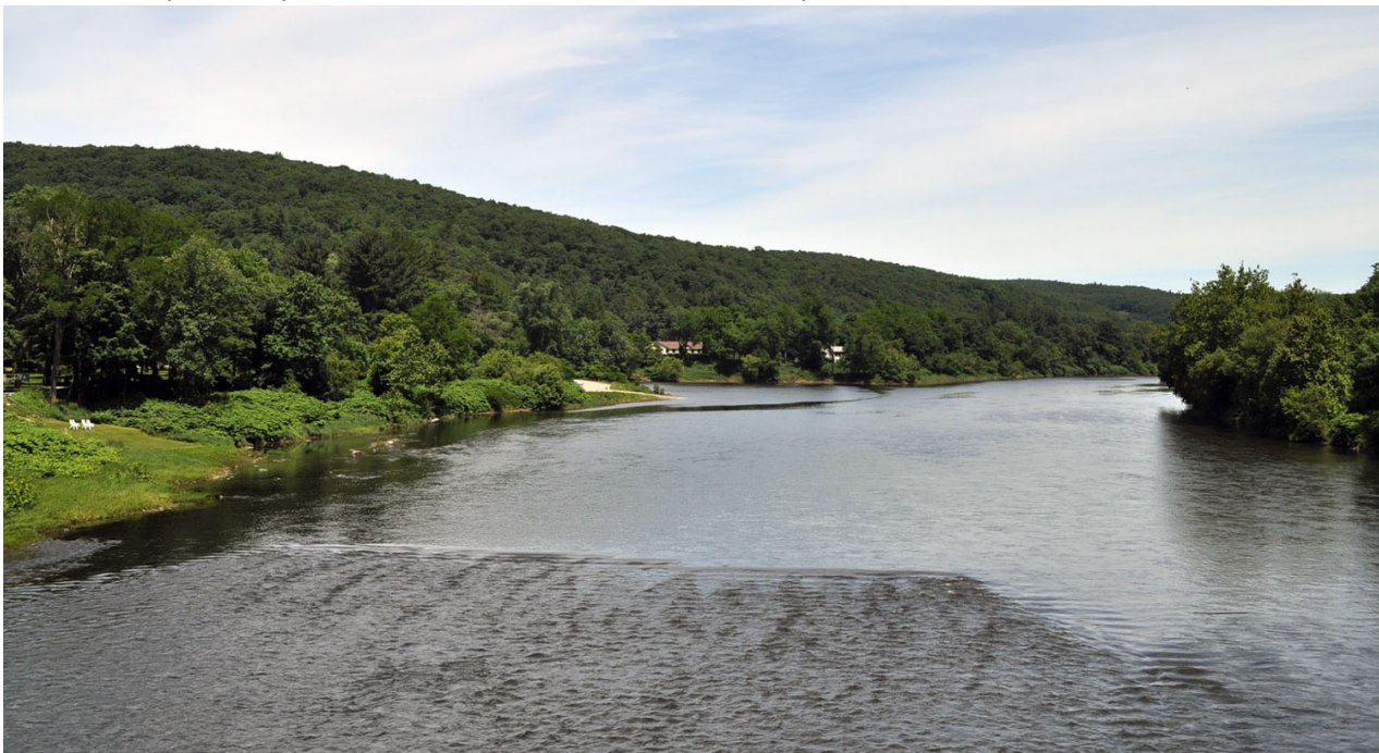
Figure 24. View of the Upper Delaware River valley, looking north from the middle of Roebling's Delaware Aqueduct. The ripples in the water are caused by the remnants of a slackwater dam. The Lackawaxen River is visible upstream. (OCLP 2015, DSC_0418)
