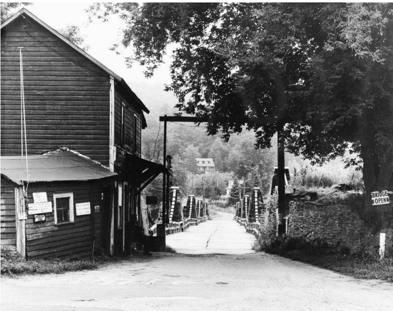
Figure 21. View looking west at tollhouse and former aqueduct, c.1968. The structure's decking and railings are in poor condition. The toll gate is a simple hinged horizontal crossbar (shown here in a raised position). (HAER PA-1, 1968, 140680pv)
