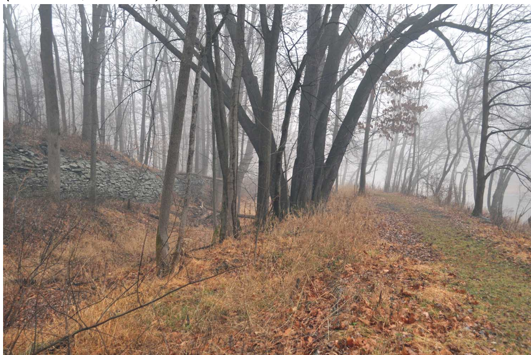
Figure 32. View looking south-southeast from the old canal towpath at the old canal prism and some of the new canal towpath stone wall. (OCLP 2013, DSC_0528)
