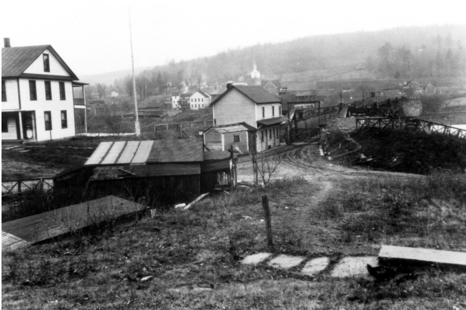
Figure 15. View of the tollhouse on the New York side of the former aqueduct, December 1923. Note the reuse of the towpath fences at image right. (Delaware and Hudson Railway Company, New York State Library)
