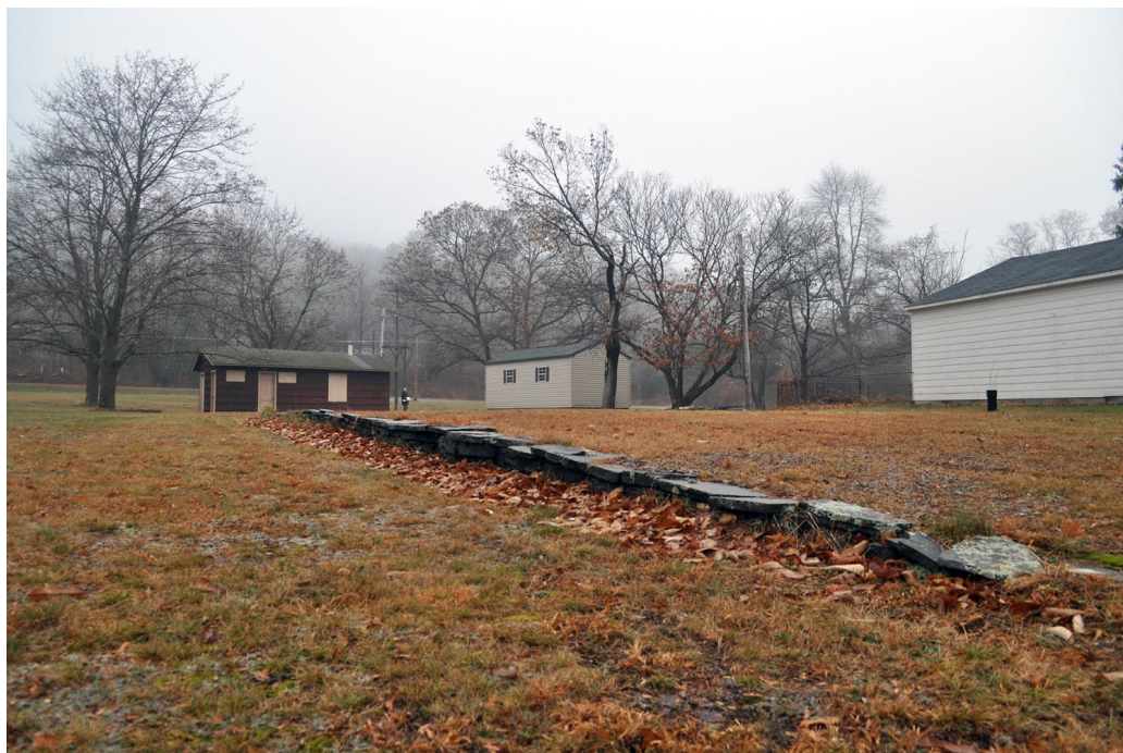
Figure 37. View looking west-northwest at the two park sheds and a low retaining wall. The building at far image right is not owned by the park. (OCLP 2013, DSC_0369)
