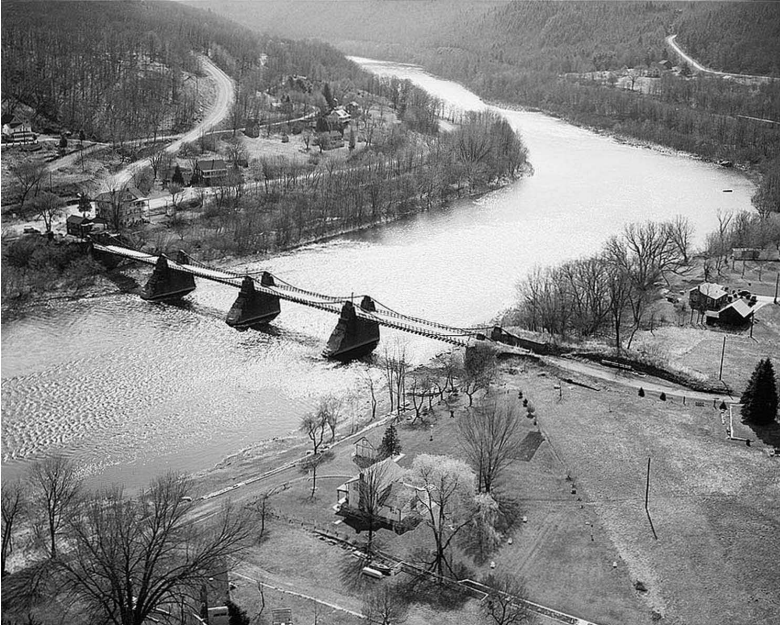
Figure 20. View looking southeast at Roebling's Delaware Aqueduct Site, c.1968. Note the poor condition of the upstream side of the aqueduct piers. On the Pennsylvania side, only a small section of towpath survives. (HAER PA-1, 1968, 140671pv)
