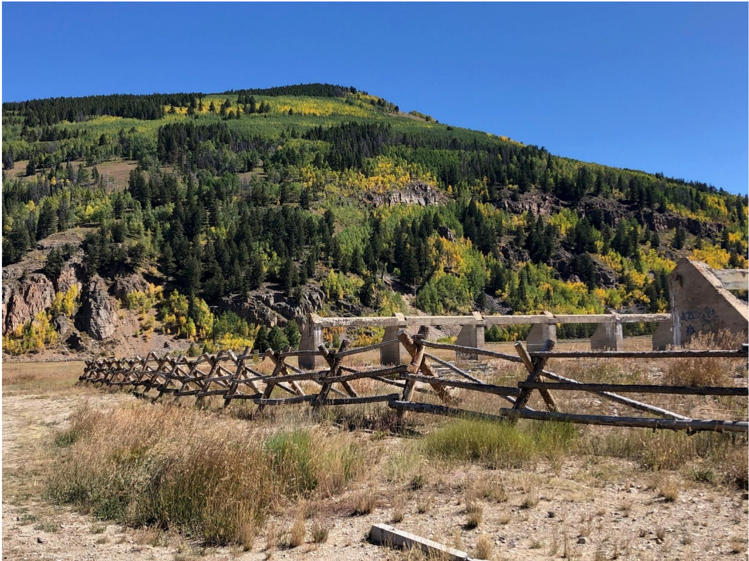
Concrete ruins of the Field House at Camp Hale, 2019
