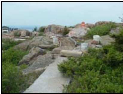
Trail construction on Cadillac Mountain
