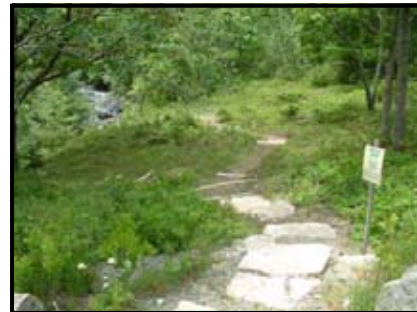
Stabilizing a steep trail path
