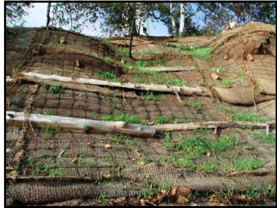
Vegetative crib wall and slope grid installed
