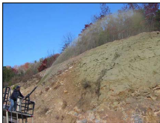
A mixture of annual and perennial grasses and native grass, wildflower, and tree seed being hydro seeded on the cut slope
