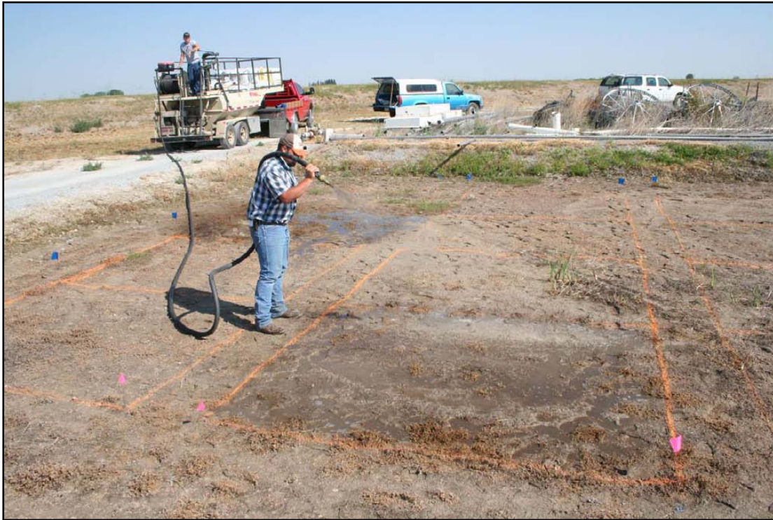
Hydroseed application of Fertil Fibers treatment.
