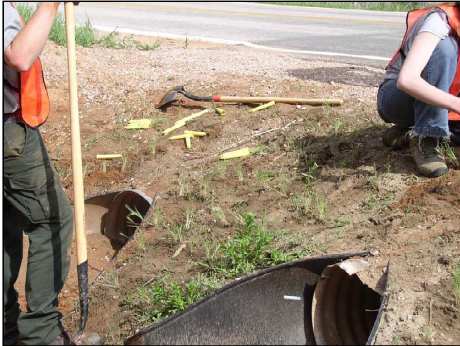
Installation of Western Wheatgrass plugs for erosion control
