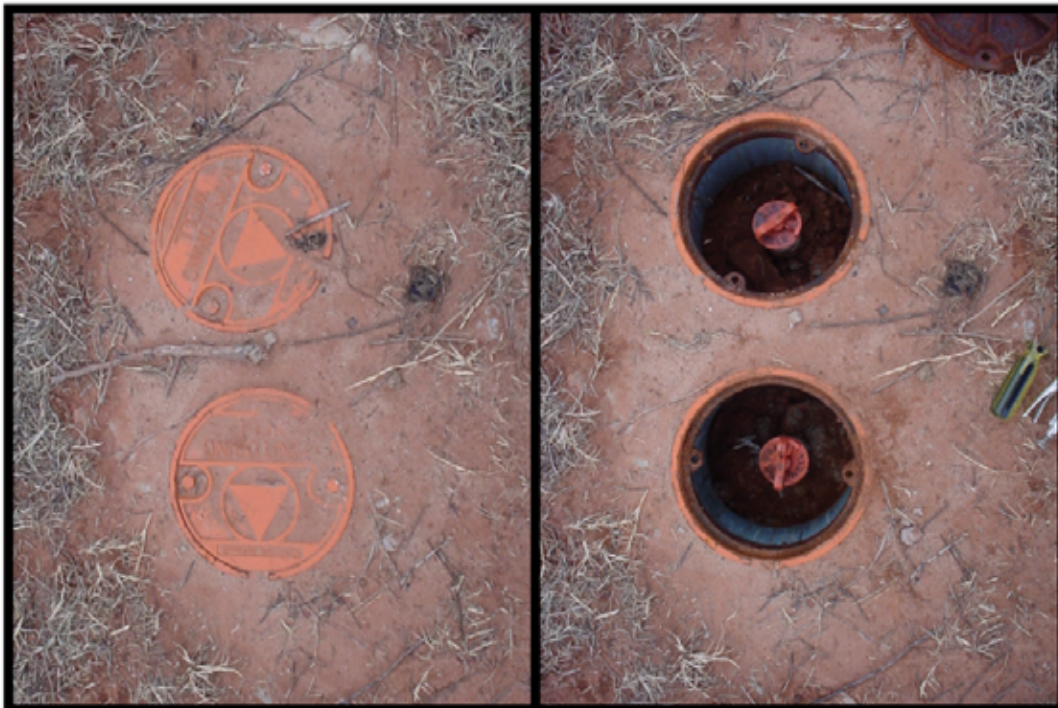
Figure 8. Photo of Wells WB-09 and WB-10 showing ground-level completion well caps used to protect PVC wells (2003).
