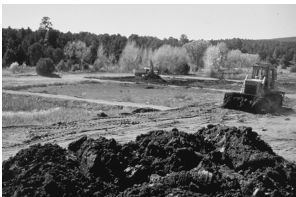
Reservoirs are being removed and the floodplain is being reshaped to create a functional wetland-riparian ecosystem.
