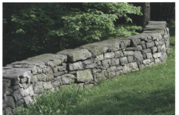
The section of the Platt Wall next to the Weir House.
