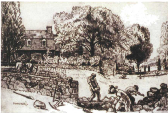
Joe Knoche builds a Stone Wall by Mahonri Young shows the construction of Cora’s “Great Wall.”
