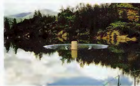
Whiskeytown's glory hole is an overflow spillway.
