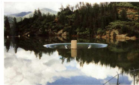
The overflow spillway is about 24 feet wide.
