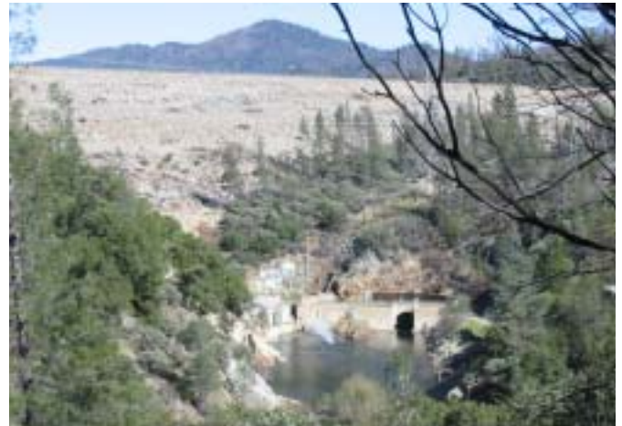
View of Whiskeytown Dam
