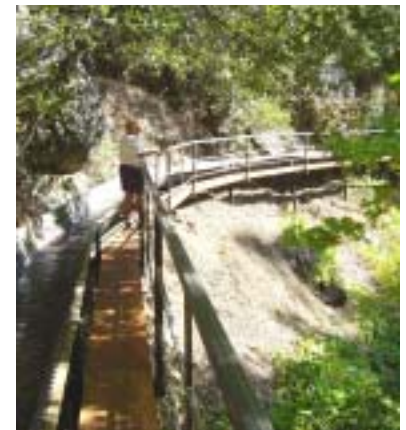
Exercise caution when traversing the trestle boardwalk
