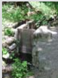
Ditch entrance gate
