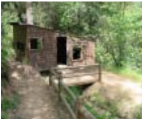
Clean out house
