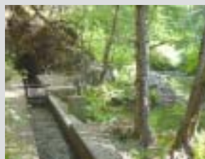
Concrete sluice discharges into short tunnel.
