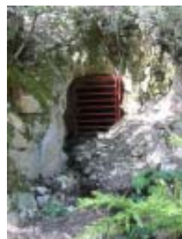
Bat gate at mine opening.
