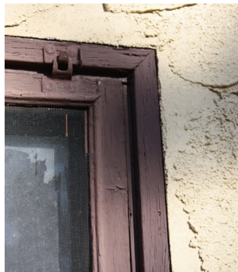
Figure W5. Photograph and detail of original top-hung wood screened sash at original wood Window 107. (SRJA 2015)
