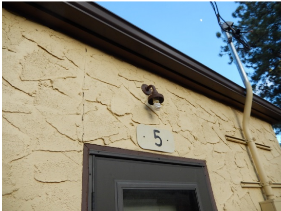
Figure X27. West Elevation detail at door. (SRJA 2015)
