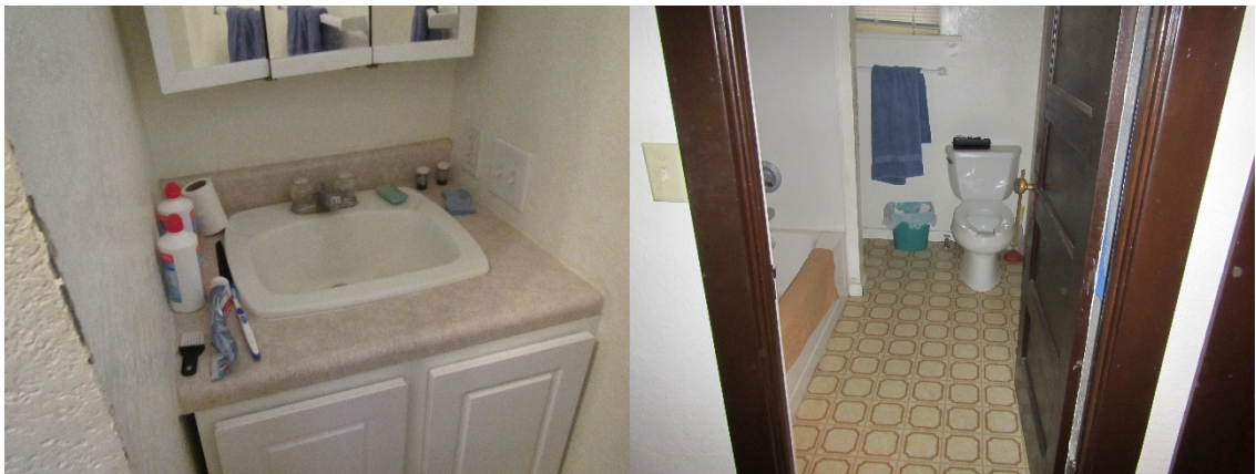
Figure P11. Lavatory and water closet in Bathroom 108. (HEI 2015)
