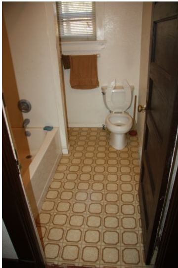
Figure 1-42. Bathroom 108 Looking north. (SRJA 2014)
