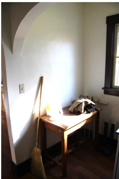
Figure 1-20. Mud Room 103 east wall. (SRJA 2014)
