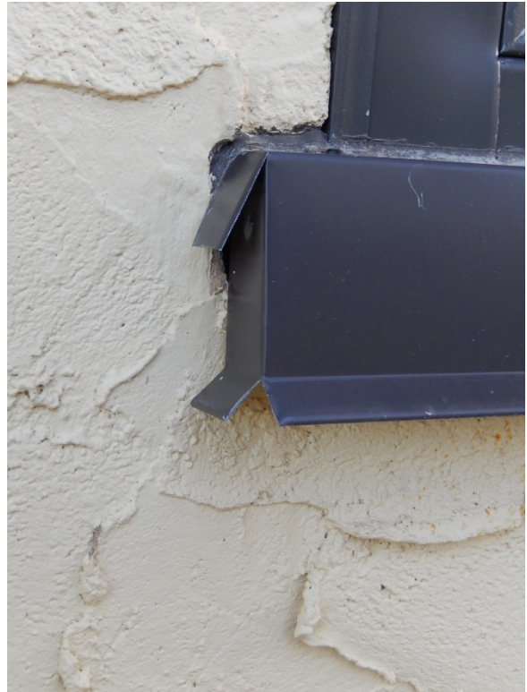
Figure X33. North Elevation Window 110 sill panning detail. (SRJA 2015)
