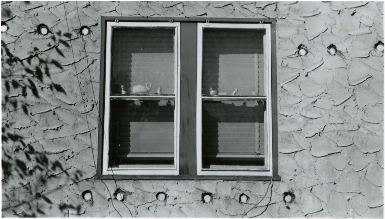
Figure 18. HS-05, ca.1952. Holes bored through stucco for insulation at Window 104. (WICA 4273)
