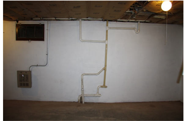
Figure B-5. Basement Looking south. (SRJA 2014)
