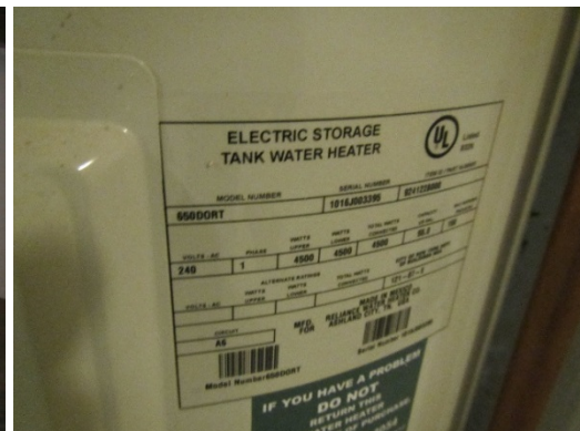
Figure P05. Domestic electric water heater in Basement 001. (HEI 2015)
