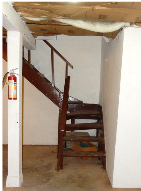
Figure 1-29. Stair 104 from basement. (SRJA 2015)
