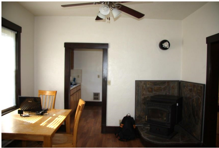
Figure 1-15. Dining Room 101 east wall. Note the flue is disconnected from the pellet stove and is covered. (SRJA 2014)
