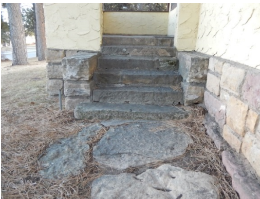
Figure X4. Front porch stone steps. (SRJA 2015)
