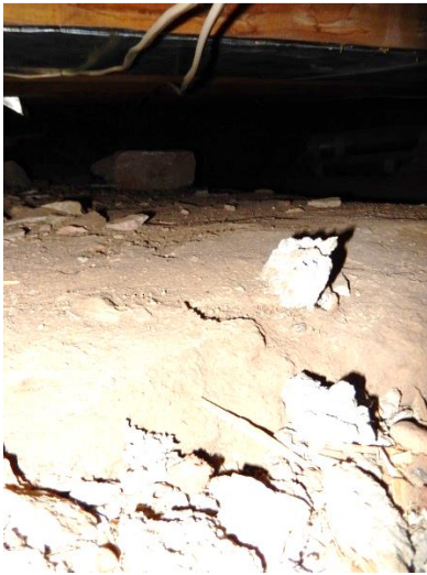
Figure B-9. Crawl Space 002 Looking east. (SRJA 2014)
