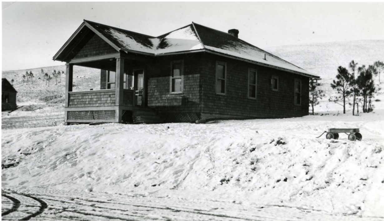
Figure 12. HS-05, ca.1935, looking southwest. (WICA 4732)
