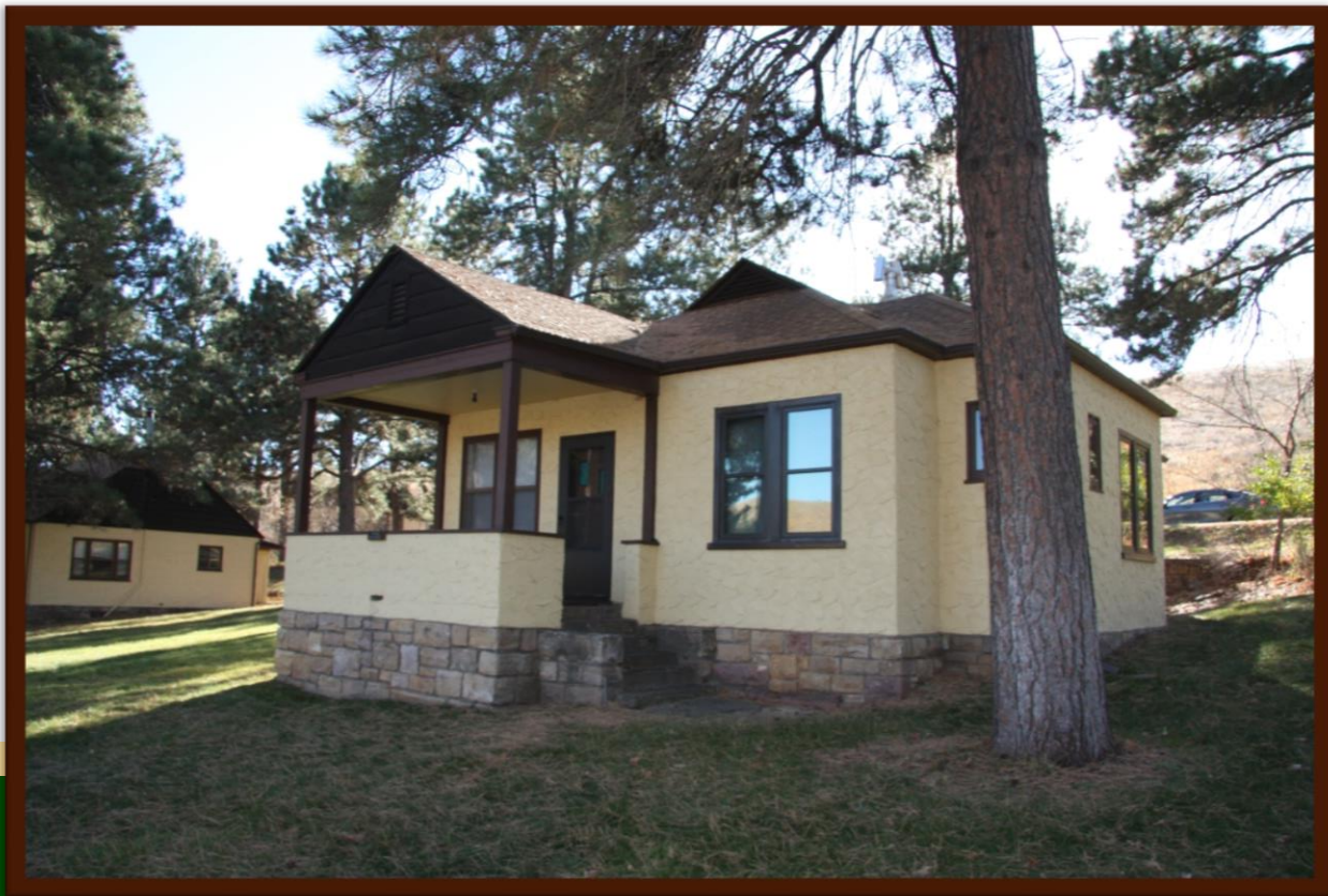
HS-05 East Elevation. (SRJA 2014)
