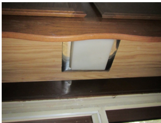
Figure E09. Light fixture located above the sink in Kitchen 102. (HEI 2015)
