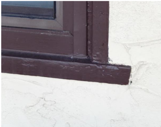
Figure W3. Detail typical mulled window with original wood trim and storm window at Window 102. (SRJA 2015)
