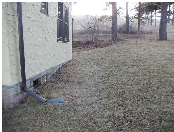
Figure X31. North Elevation of house looking west at north-south grad cross-slope towards house. (SRJA 2015)
