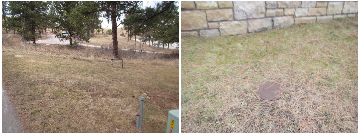
Figure P01. Shutoff valves, irrigation vacuum breaker, and sanitary sewer cleanout. (HEI 2015)
