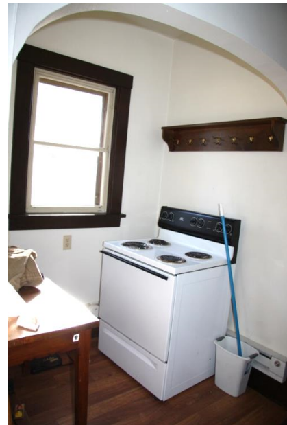
Figure 1-21. Mud Room 103 south and west walls. (SRJA 2014)
