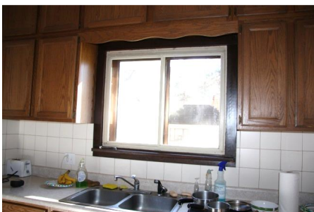
Figure 1-17. Kitchen 102 south wall looking at Window 105. (SRJA 2014)
