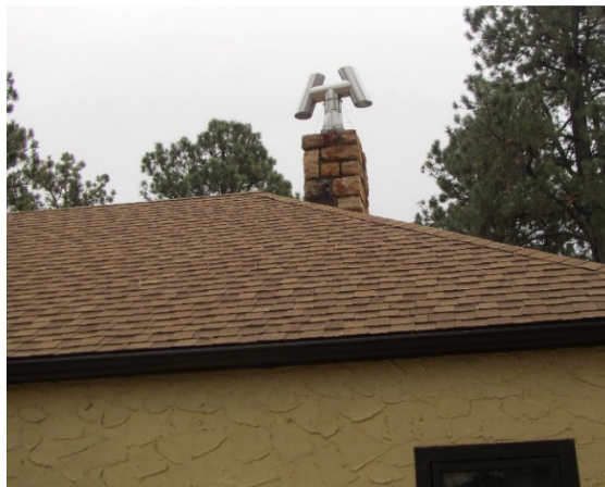
Figure M04. Pellet burner flue termination. (HEI 2015)
