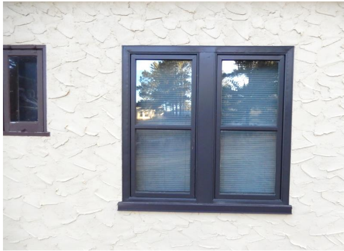
Figure W9. Detail of historic wood Window 114 on the left adjacent to replacement aluminum casement Window 113 with metal panning over the trim. Note the metal trim is much thicker at the side and at the sill. (SRJA 2015)
