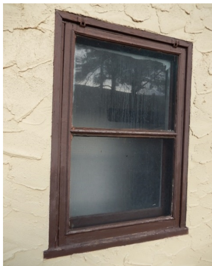
Figure W5. Photograph and detail of original top-hung wood screened sash at original wood Window 107. (SRJA 2015)
