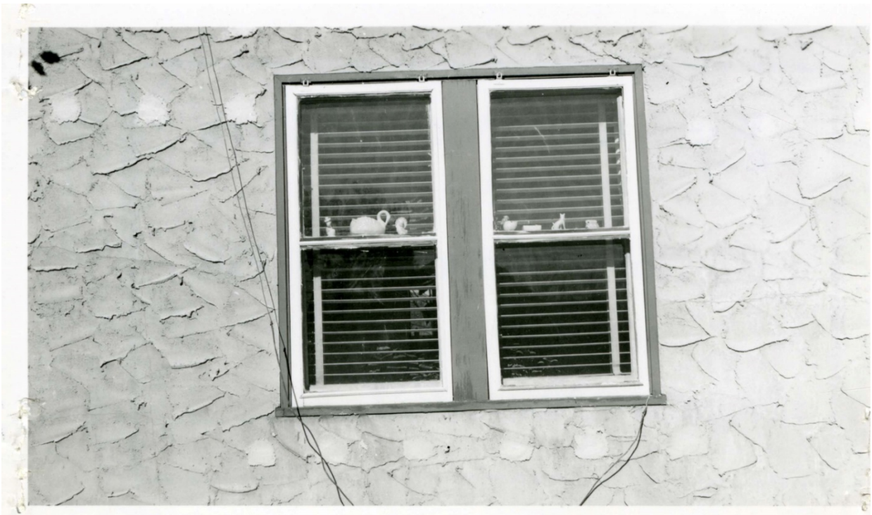
Figure 19. HS-05, ca.1952. Same view, after stucco repair from insulation installation. Figure 20. (WICA 4731)
