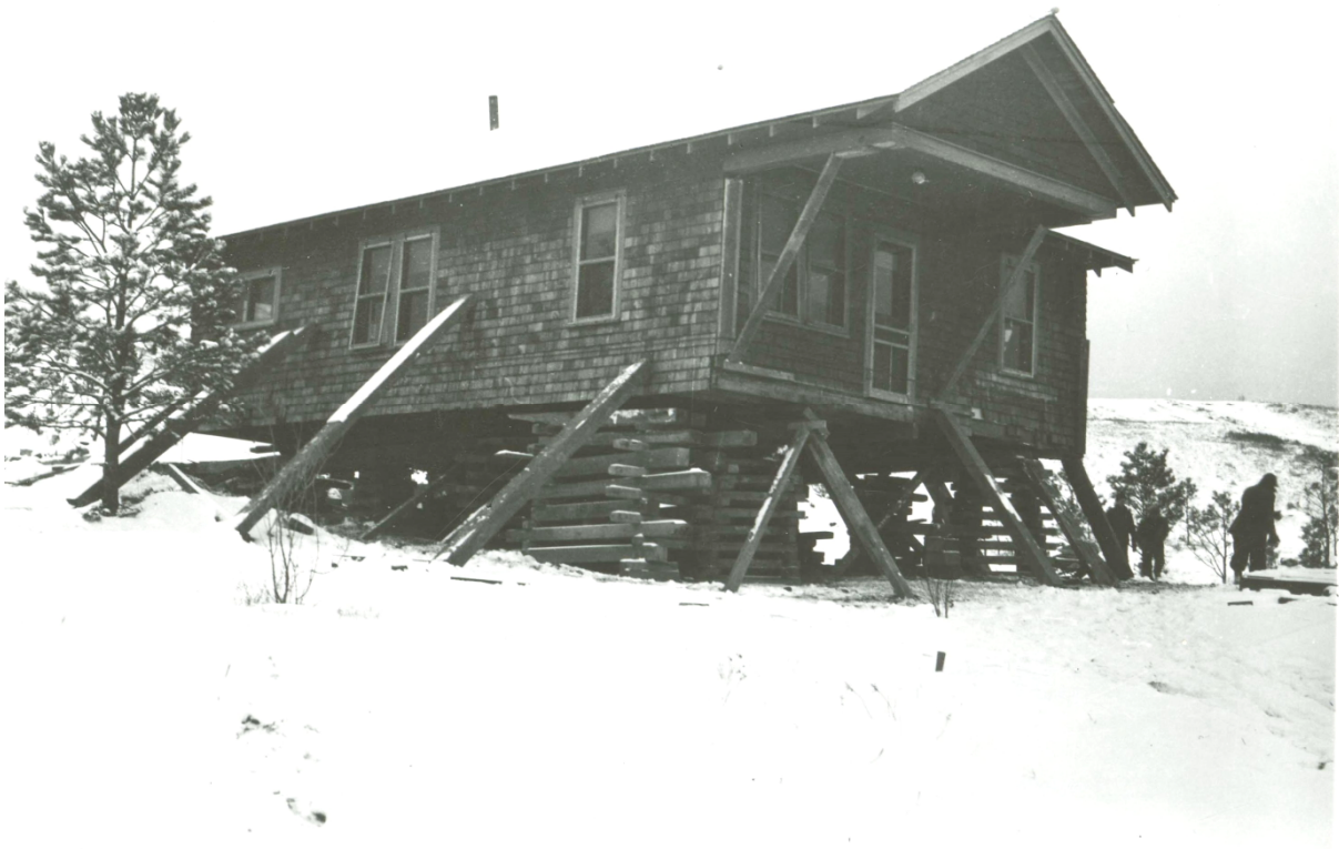
Figure 13. HS-05, ca.1935, looking north. The building has been lifted and shored to prepare for its move to a new site. (WICA 4274)
