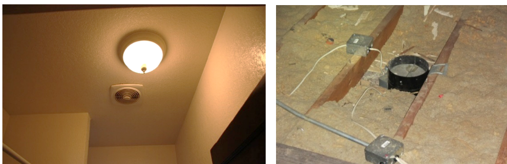
Figure M08. Bathroom – 108, Exhaust fan and termination. (HEI 2015)
