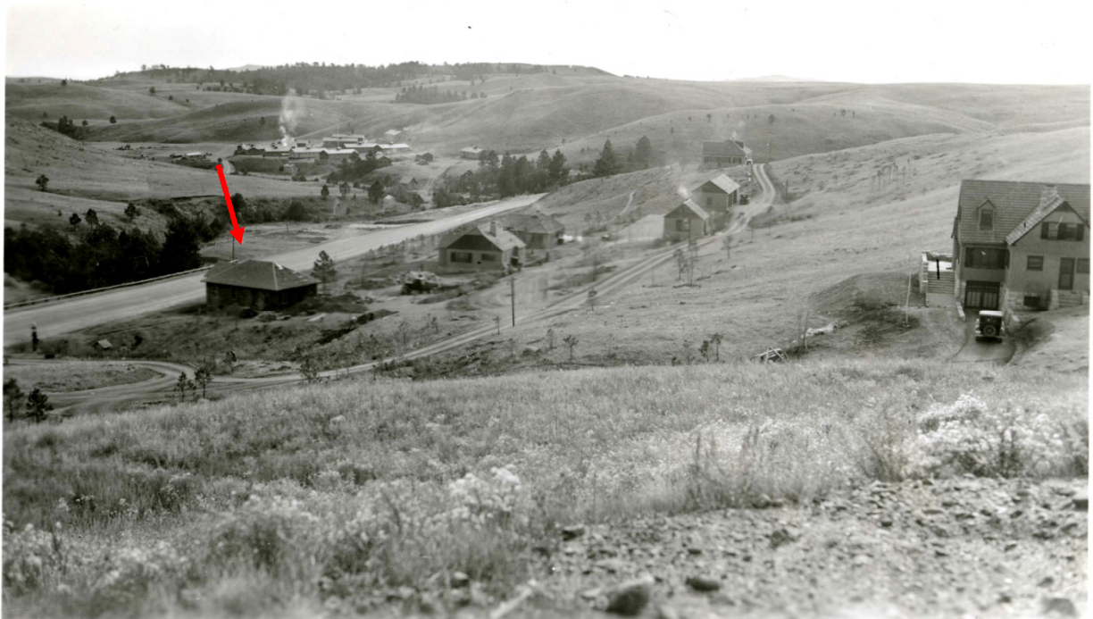
Figure 11. Nov. 10, 1934, looking south. HS-05 shortly before it was moved to its present location. (WICA 4335)
