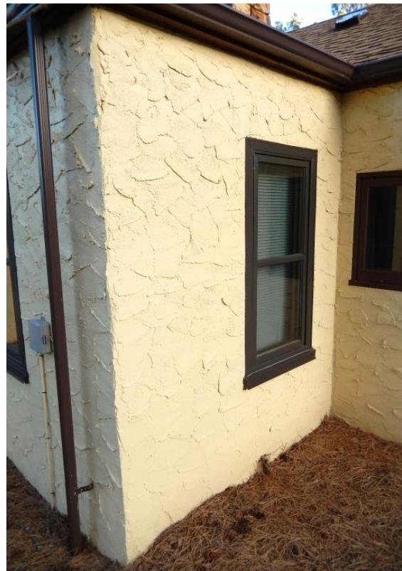
Figure X29. West Elevation Window 109. (SRJA 2015)
