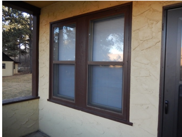
Figure W2. Typical mulled Window 102 with original wood trim and metal storm window. (SRJA 2015)
