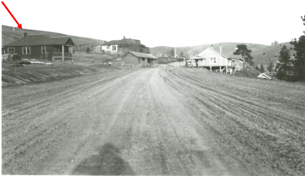
Figure 6. Headquarters area, ca.1926, looking north. (WICA 4163)
