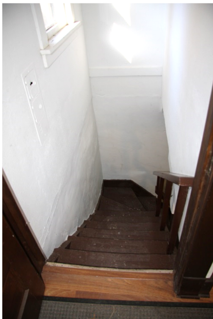
Figure 1-24. Stair 104 Looking north. (SRJA 2014)
