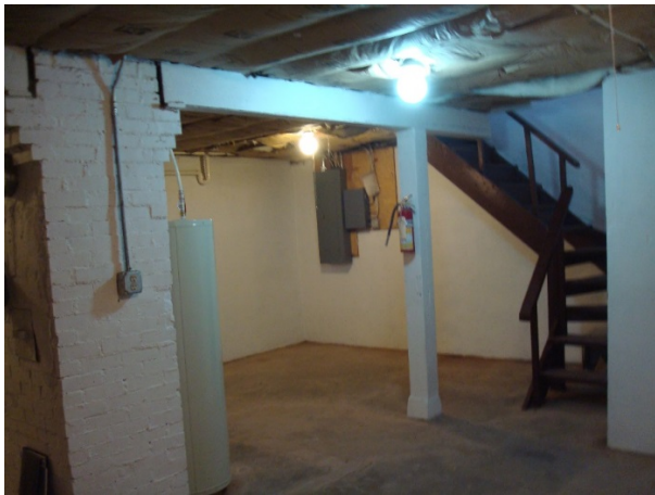
Figure S2. West girder in basement. (SEA 2015)
