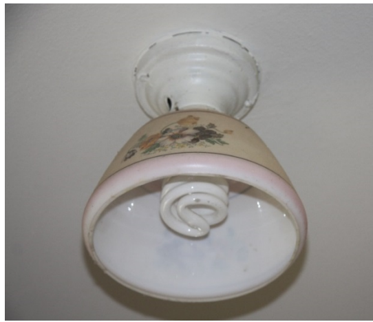
Figure E10. Light fixture located above the laundry area in Mud Room 103. (SRJA 2014)
