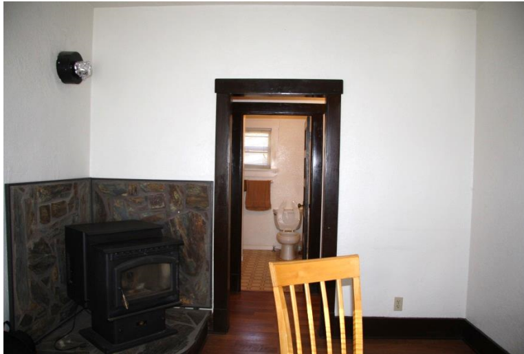
Figure 1-12. Dining Room 101 north wall. (SRJA 2014)
