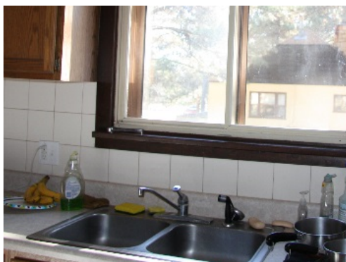
Figure P09. Stainless steel two-compartment sink in Kitchen 104. (HEI 2015)
