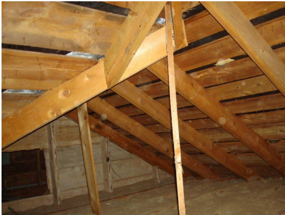
Figure S8. 1x members supporting hip rafter. (SEA 2015)
