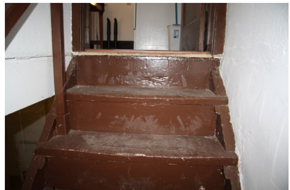
Figure 1-25. Stair 104 Detail looking south. (SRJA 2014)
