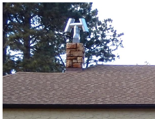
Figure X20. South Elevation chimney detail. (SRJA 2015)
