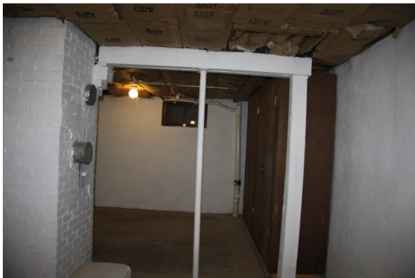
Figure B-2. Basement Looking north. (SRJA 2014)
