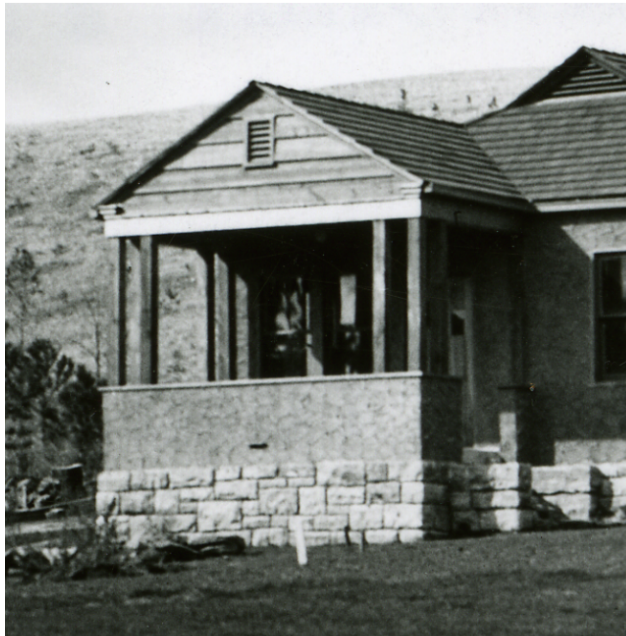
Figure X2. Detail of HS-05 front porch, 1935, May 1. Note the double columns on the porch. (WICA 4259.)
