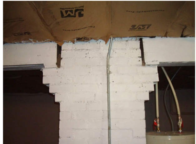
Figure S3. Girders bearing on chimney haunch. (SEA 2015)
