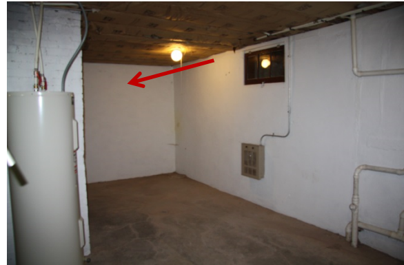
Figure B-10. Basement 001 Looking south and east. The red arrow points to where there used to be a larger crawl space access that has been infilled. (SRJA 2014)
