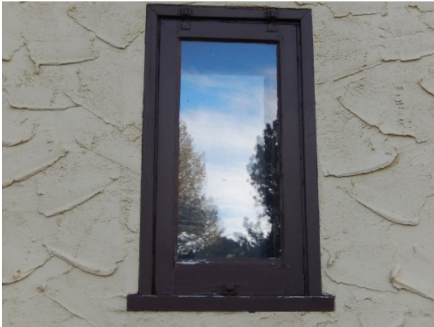
Figure W6. Detail of original top-hung storm sash at original wood Window 114. (SRJA 2015)
