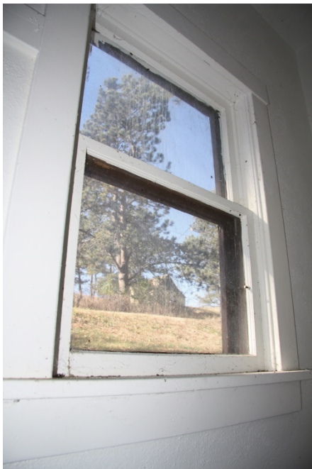
Figure 1-26. Stair 104 Window 107. One of two original 1/1 double-hung wood windows in the house. (SRJA 2014)
