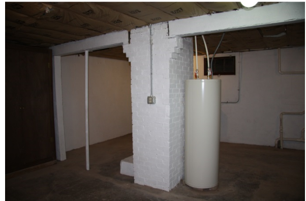
Figure B-4. Basement Looking southeast. (SRJA 2014)
