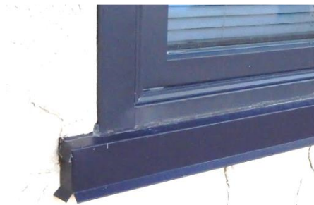
Figure W10. Detail of aluminum replacement Window 113 metal trim and sill panning. (SRJA 2015)
