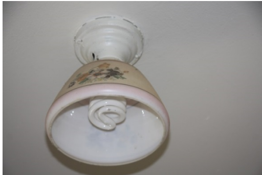
Figure 1-23. Mud Room 103 light fixture detail. (SRJA 2014)
