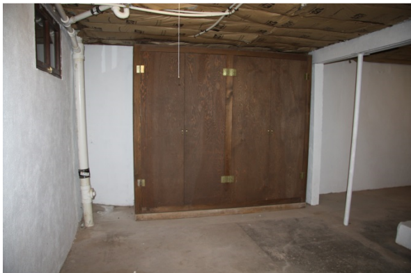
Figure B-3. Basement Looking east. (SRJA 2014)
