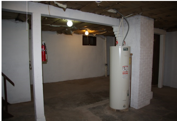
Figure B-1. Basement Looking northeast. (SRJA 2014)
