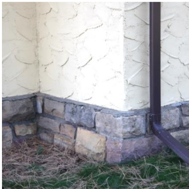
Figure X3. Northeast corner of the building. (SRJA 2014)
