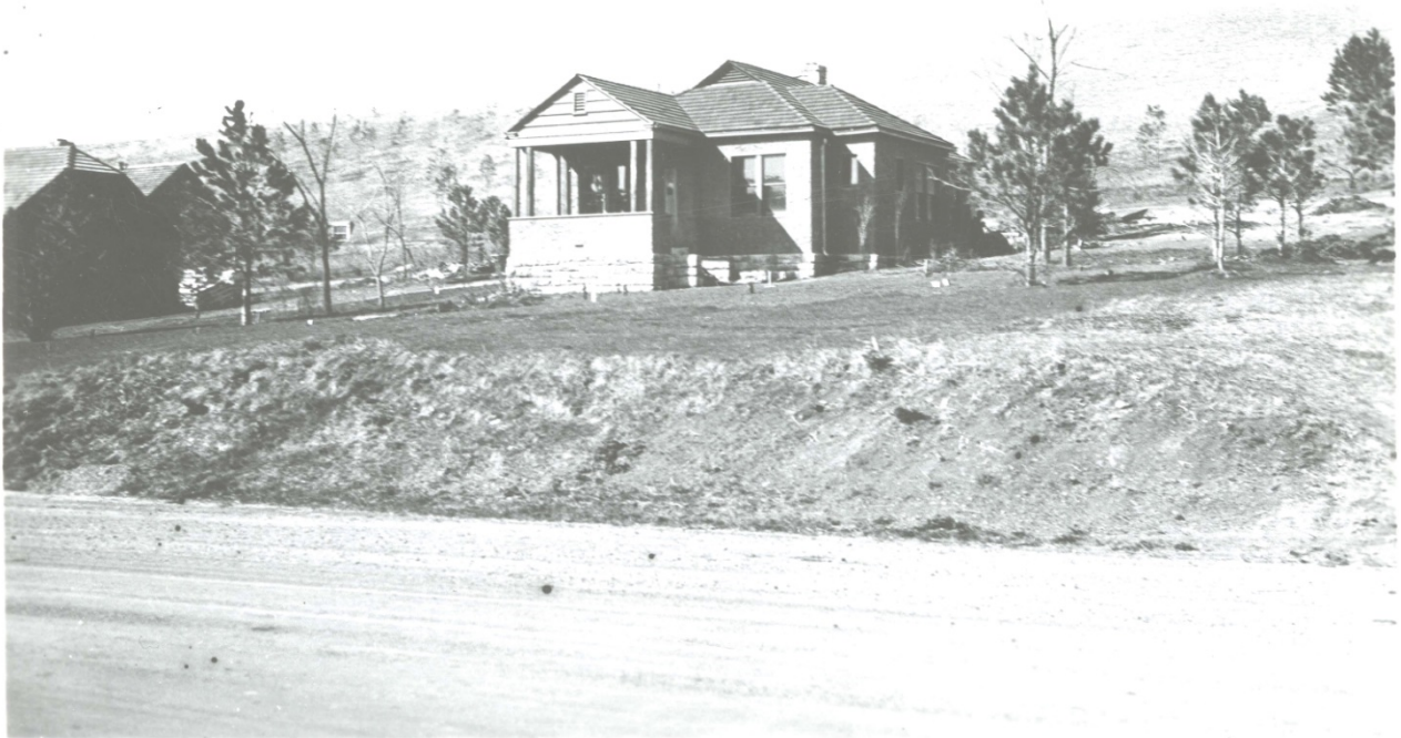
Figure 16. HS-05, ca.1935, looking southwest. (WICA 4722)
