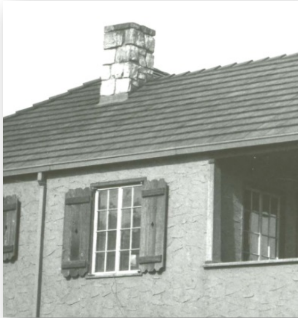
Figure W1. HS-07. ca.1940. Note the steel casement windows and the rustic board and batten shutters with the diamond silhouette design in the center. (WCNP Archive Number: WICA 4730.)
