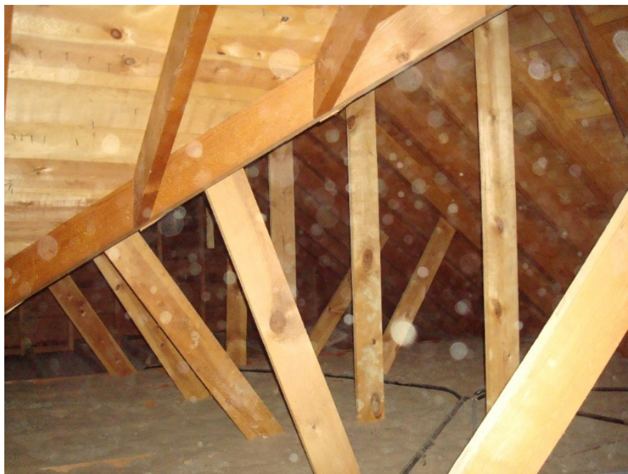
Figure S11. Roof framing, 1x6 bracing bearing on ceiling joists. (SEA 2015)
