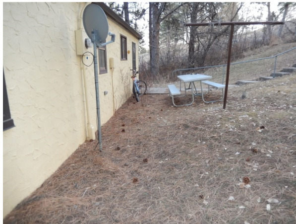
Figure X29. West Elevation grade, looking south. (SRJA 2015)
