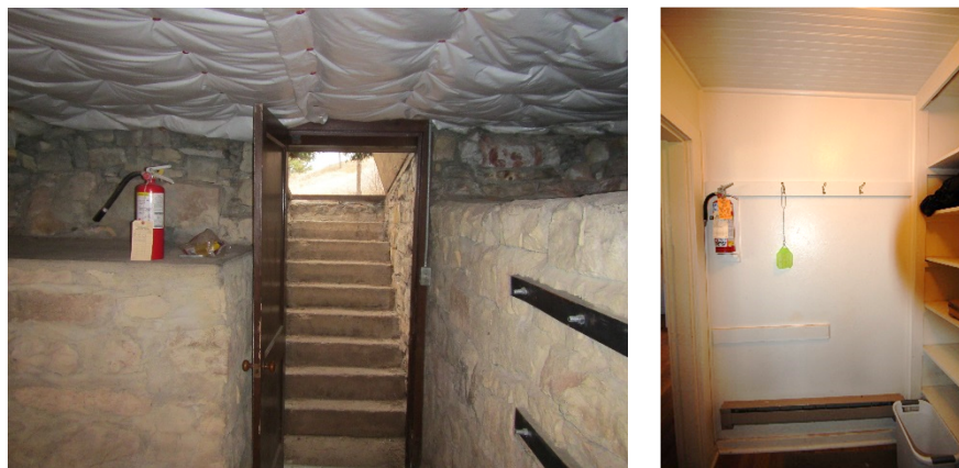
Figure F01. Fire extinguishers. (Basement 001-Left, West Entry 103-Right) (HEI 2015-Left, SRJA-Right)
