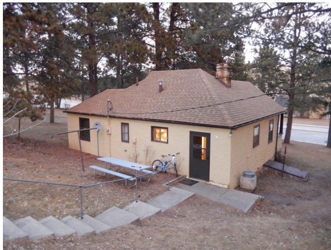
Figure R1. West-facing roof. (SRJA 2015)
