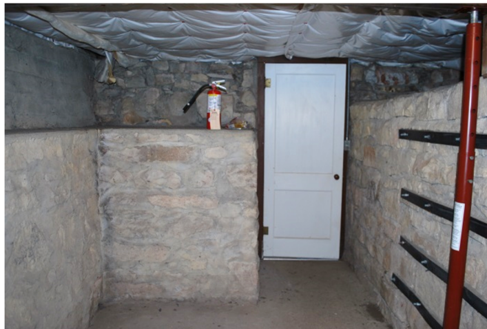
Figure B-2. Basement Room 001 Looking south. (SRJA 2014)
