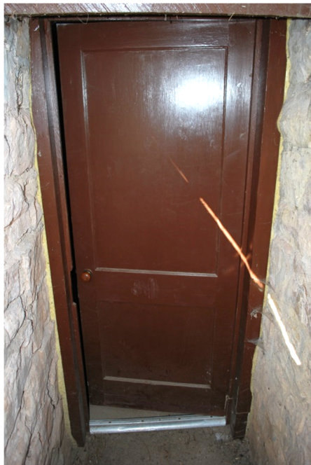
Figure B-1. Basement Door 001/1 from the bulkhead. (SRJA 2014)
