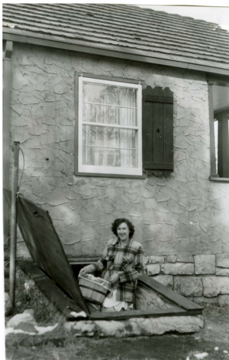
Figure 15. HS-07, ca.1952, looking north. The counterweight post to the left of the bulkhead still exists. (WICA 6853)
