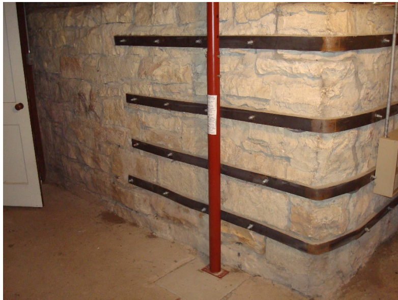
Figure S2. Repair to existing stone retaining wall looking southwest. (SEA 2015)
