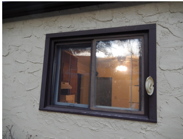
Figure X32. West Elevation Window 105. (SRJA 2015)
