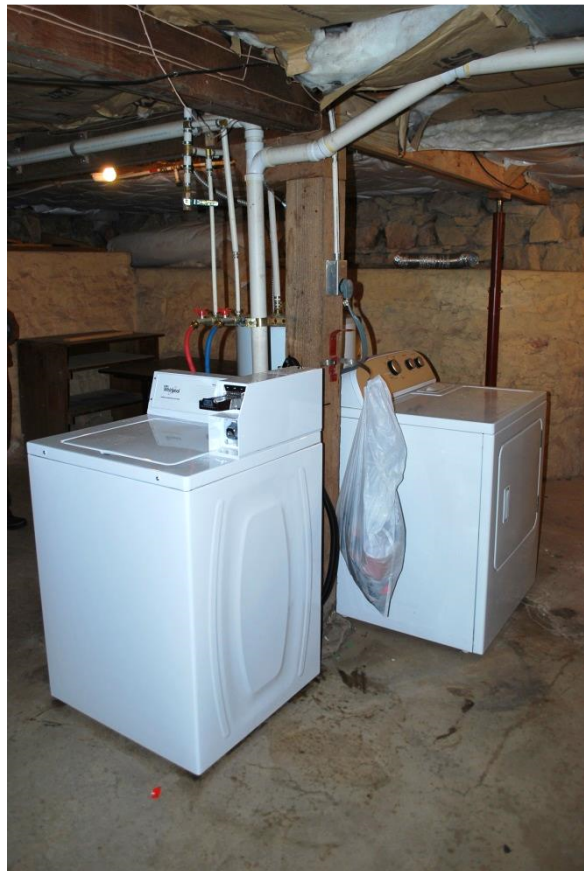
Figure B-8. Basement Room 001 Looking northeast at center post. (SRJA 2014)
