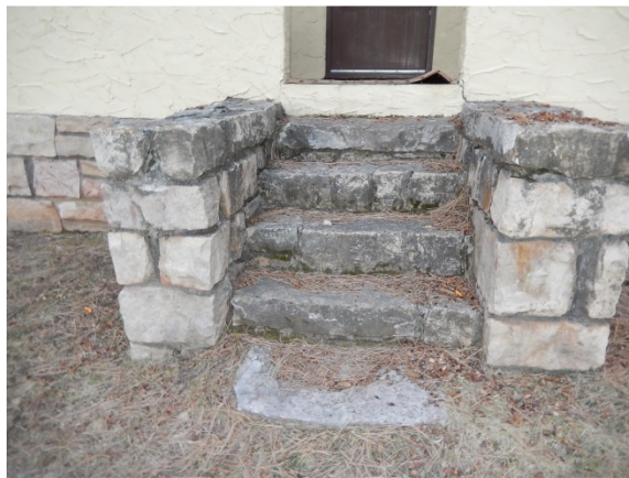
Figure X8. Porch Steps – East Elevation. (SRJA 2015)
