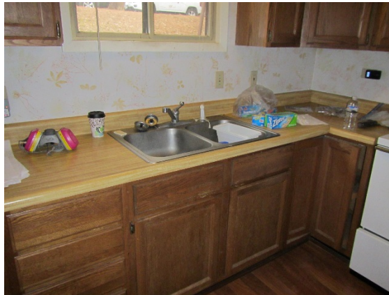
Figure P07. Stainless steel two-compartment sink in Kitchen 104. (HEI 2015)
