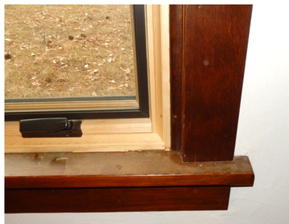
Figure F-3. Typical millwork profiles – Flat stock window stool and apron with eased edges. (SRJA 2015)
