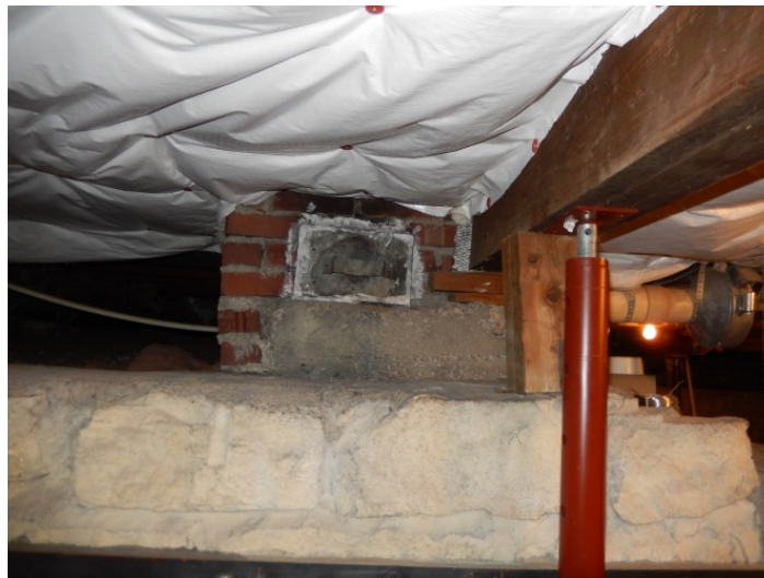
Figure B-4. Basement Room 001 Looking west at chimney. (SRJA 2015)
