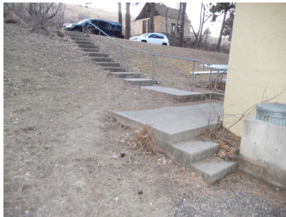
Figure X28. West Elevation steps and grade, looking northwest. (SRJA 2015)
