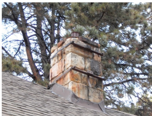
Figure X26. Chimney detail. (SRJA 2015)
