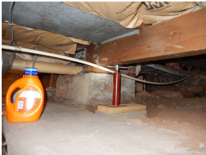
Figure B-6. Basement Room 001 Looking southeast at chimney. (SRJA 2015)
