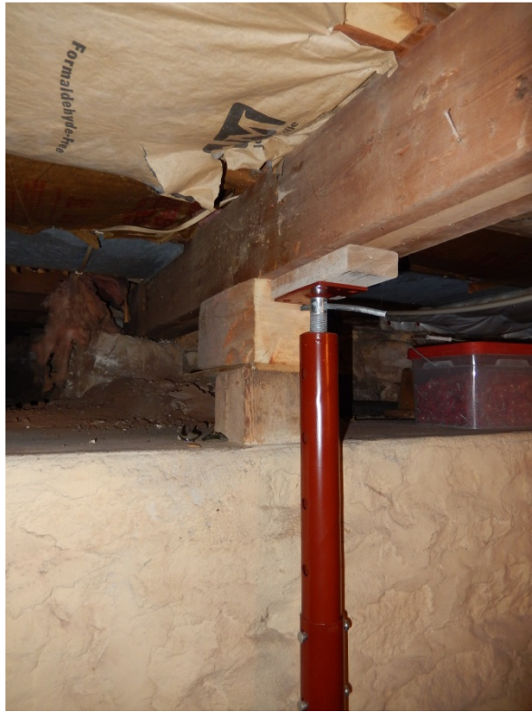
Figure B-15. Basement Room 001 Looking at north side of beam. (SRJA 2015)
