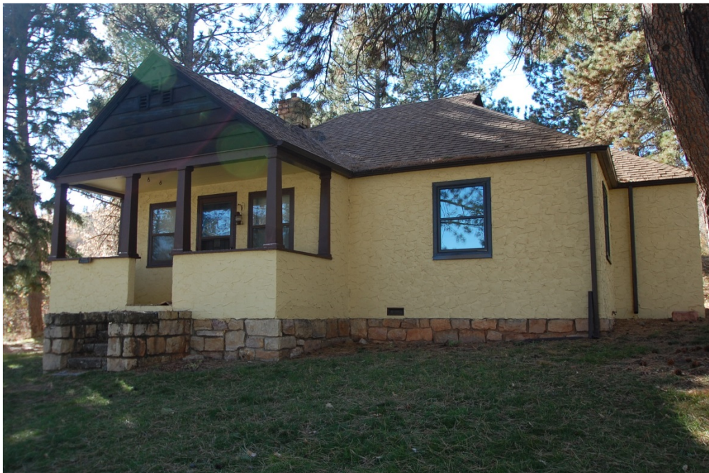
Figure X1. East Elevation. Note at the north section, the grade is above the top of the stone foundation. (SRJA 2014)
