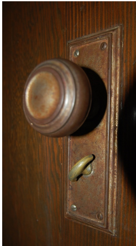
Figure 1-22. Bathroom 104 Hardware detail. (SRJA 2014)
