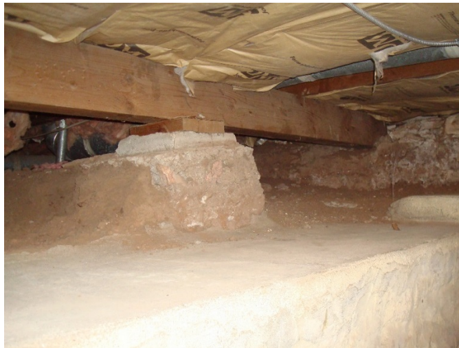
Figure S5. Girder support on original crawl space footing. (SEA 2015)
