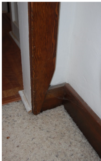
Figure 1-7. Living Room 100 Detail of millwork anomaly in the northwest corner of the room. Perhaps there was once a furnace damper in this location. (SRJA 2014)
