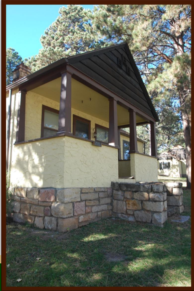
HS-07 East Elevation. (SRJA 2014)
