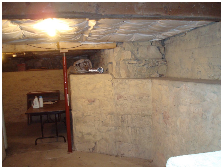
Figure S1. Stone retaining walls looking north. (SEA 2015)
