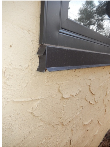
Figure W6. Window 107 on the west elevation detail. (SRJA 2015)
