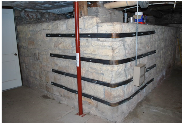
Figure B-3. Basement Room 001 Looking southwest – chimney foundation is near the corner. (SRJA 2014)
