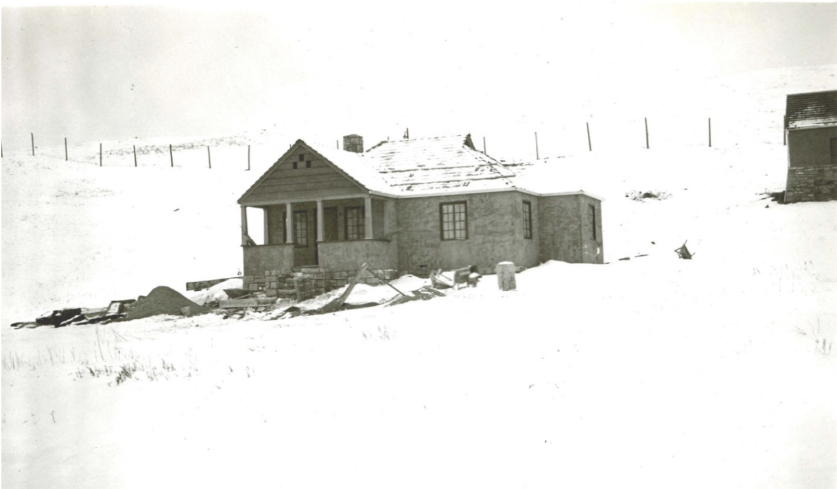
Figure 7. HS-07, 1932, Jan. 8, looking west. (WICA 4489)
