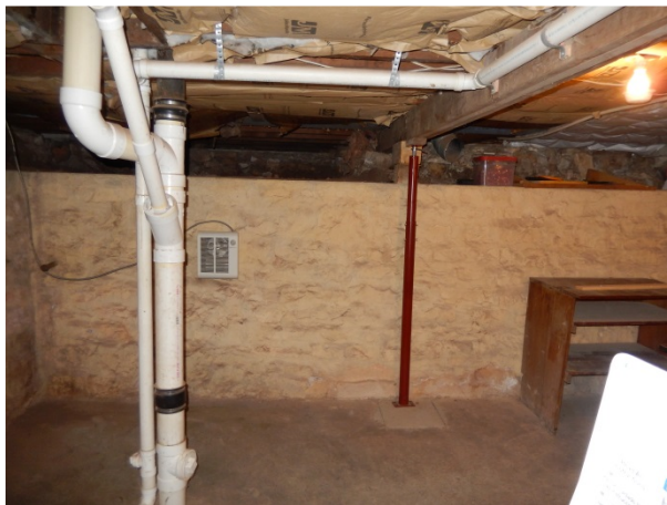
Figure B-13. Basement Room 001 Looking north towards north crawl space. (SRJA 2015)
