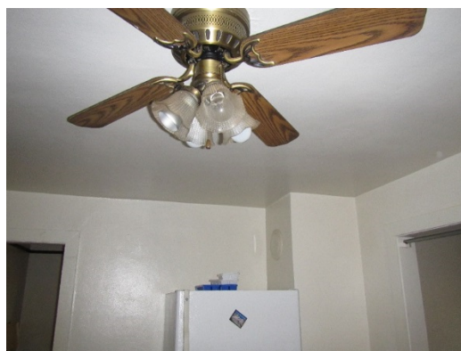
Figure E09. Ceiling fan located in Kitchen 101. (HEI 2015)
