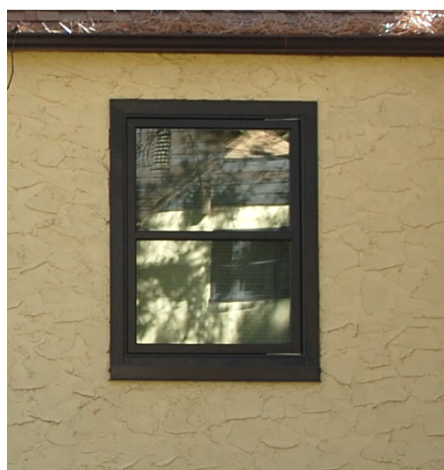
Figure W5. Window 109 on the north elevation. Aluminum replacement casement window with metal paning covering the historic trim. (SRJA 2014)
