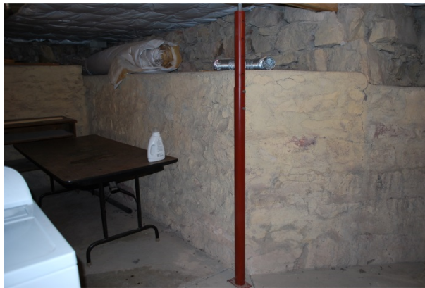
Figure B-17. Basement Room 001 Looking northeast. (SRJA 2014)
