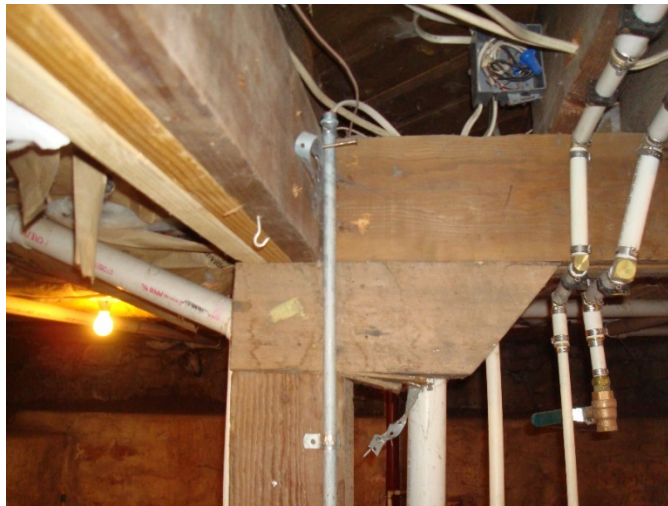
Figure S7. Corbel support of wood girder looking west. (SEA 2014)
