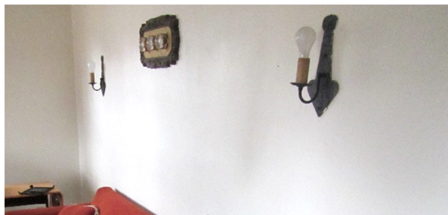
Figure E08. Historic light fixtures located in Living Room 100. (HEI 2015)
