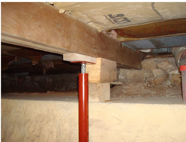
Figure S8. Support of north girder at west end looking north. (SEA 2015)
