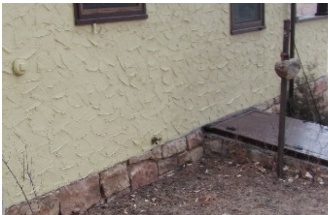
Figure P02. Wall hydrant. (HEI 2015)
