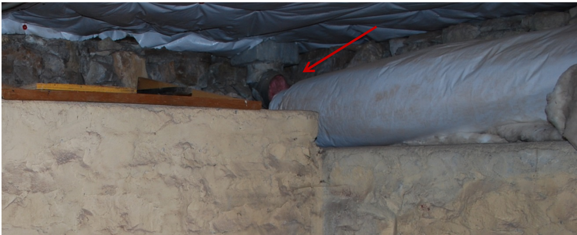
Figure B-16. Basement Room 001 Looking northeast at a sample of abandoned ductwork. (SRJA 2015)
