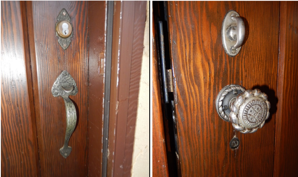
Figure X17. Front Door 100/1 hardware detail. (SRJA 2015)
