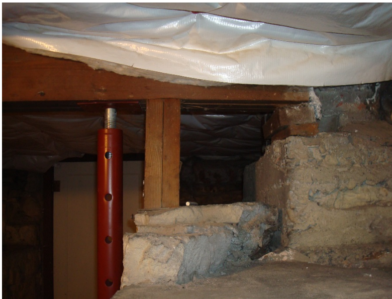
Figure S3. Room 001 girder support, east side of chimney looking south. (SEA 2015)
