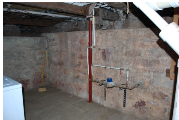
Figure B-11. Basement Room 001 Looking at west wall. (SRJA 2014)
