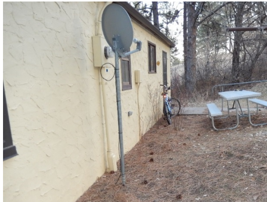
Figure E15. Telephone service located on the west exterior wall. TV satellite antenna located the west of the house. (SRJA 2015)
