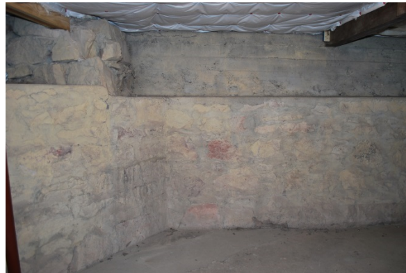
Figure B-18. Basement Room 001 Looking east at stone retaining walls and concrete porch foundation wall above. (SRJA 2014)
