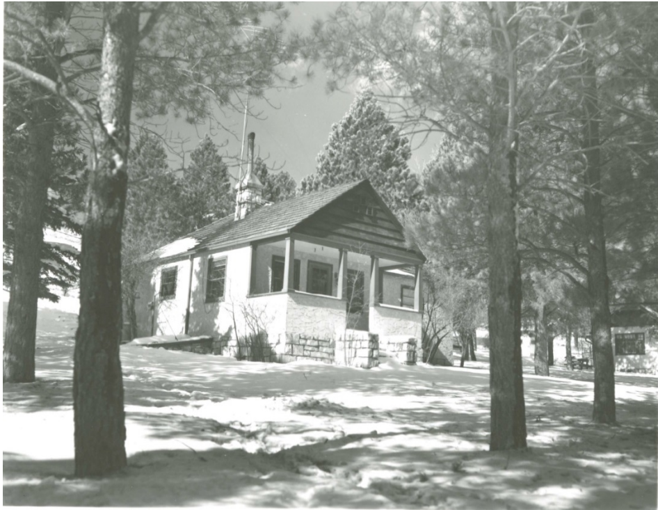
Figure 18. HS-07, ca.1969, looking west. (WICA 6706)
