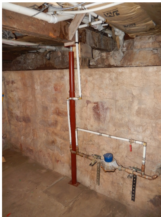
Figure S6. Girder support on steel post along east wall. Note the concrete many indicate there is a footing in this location. (SEA 2015)
