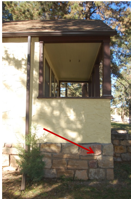
Figure X10. Porch - South Elevation. (SRJA 2014)
