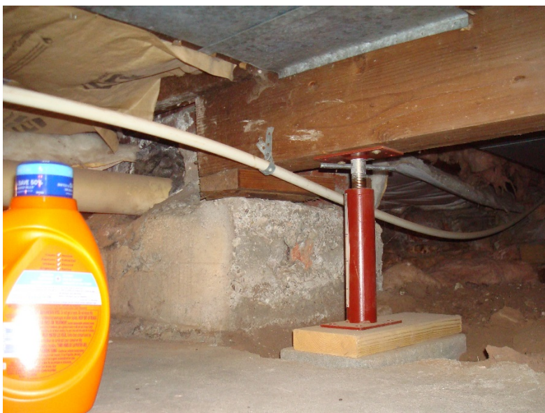
Figure S4. Girder support west side of chimney looking southeast. (SEA 2015)
