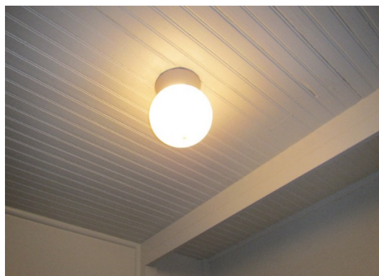
Figure E12. Light fixture located in West Entry 103 and Hall 105. (HEI 2015)
