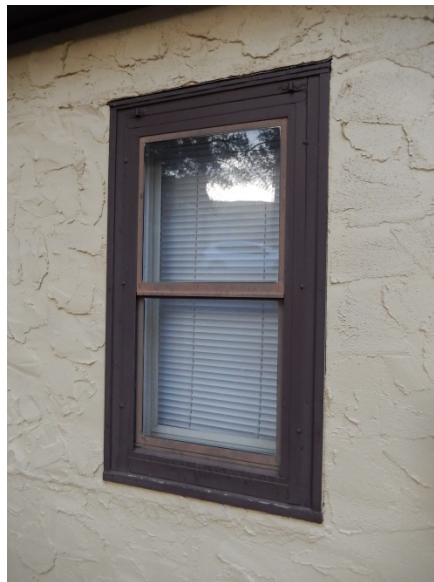
Figure W2. Window 106 on the west elevation. (SRJA 2015)
