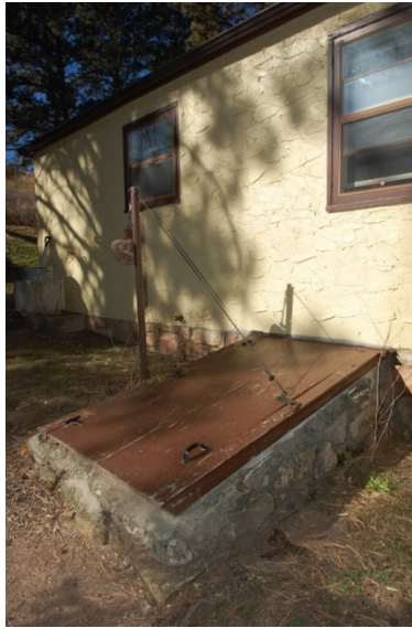
Figure X24. South Elevation bulkhead door. (SRJA 2014)
