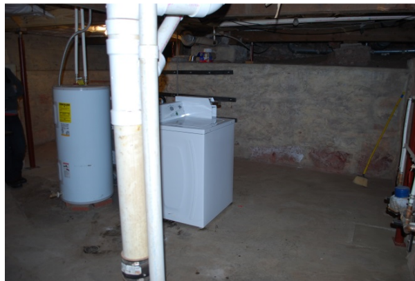
Figure B-10. Basement Room 001 Looking south. (SRJA 2014)
