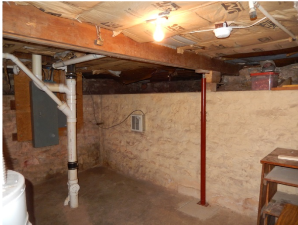
Figure B-12. Basement Room 001 Looking at west and north walls. (SRJA 2015)
