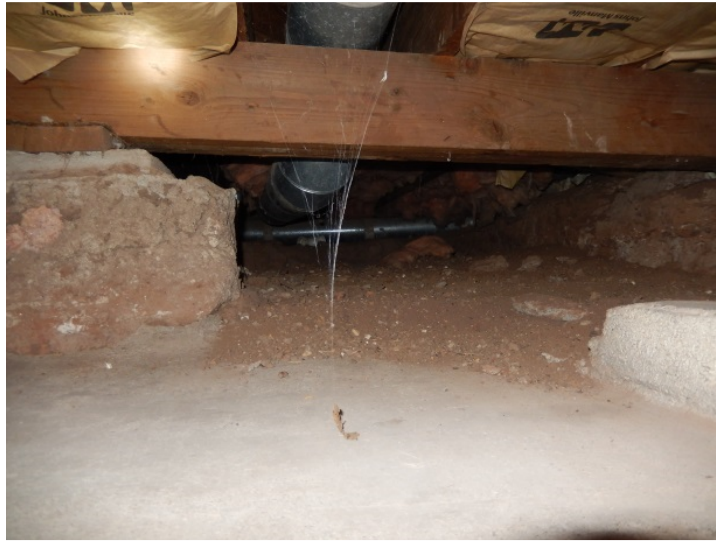
Figure B-7. Basement Room 001 Looking south into the crawl space. (SRJA 2015)
