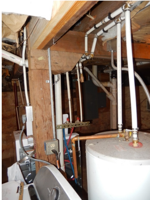
Figure B-9. Basement Room 001 Looking west at center post framing. (SRJA 2015)
