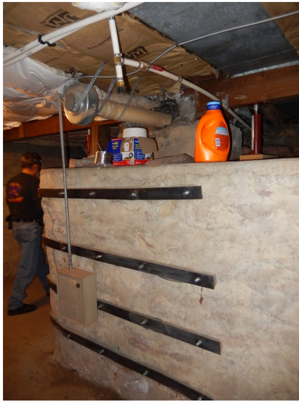
Figure B-5. Basement Room 001 Looking south at chimney. (SRJA 2015)
