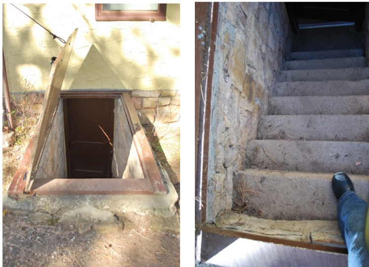
Figure X25. Basement bulkhead details. (SRJA 2015)
