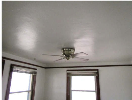
Figure E07. Ceiling fan located in Living Room 100. (HEI 2015)
