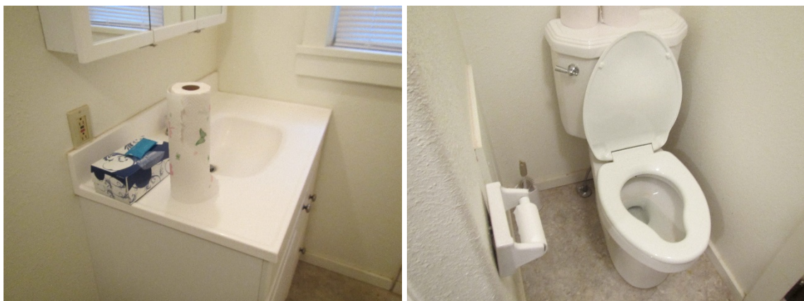
Figure P09. Lavatory and water closet in Bathroom 104. (HEI 2015)
