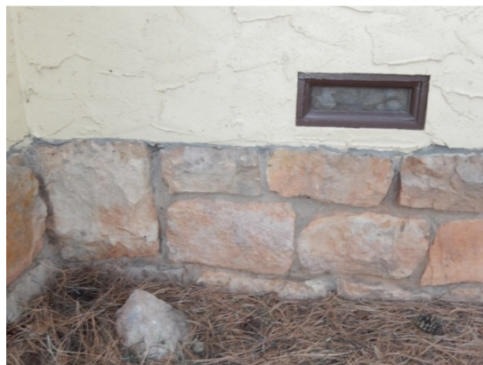
Figure X20. East elevation foundation vent detail. (SRJA 2015)
