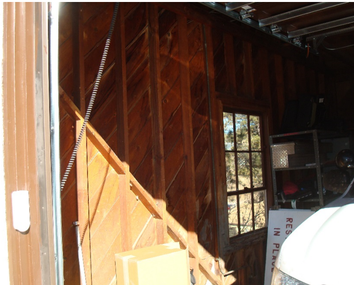
Figure. S15. Second Floor wall framing. (SEA 2015)
