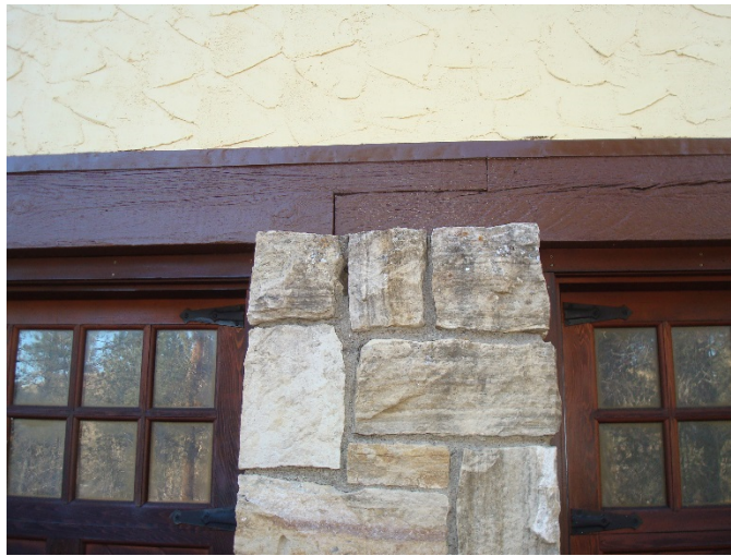
Figure S3. Girder splice over stone pilaster. (SEA 2015)
