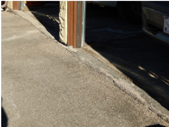
Figure X11. West Elevation detail at the garage. (SRJA 2015)
