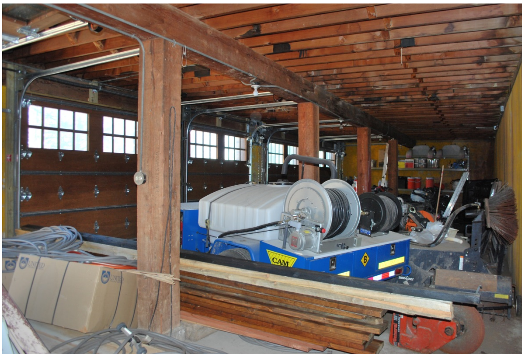
Figure 1-2. Garage 100 Looking south and east. (SRJA 2014)
