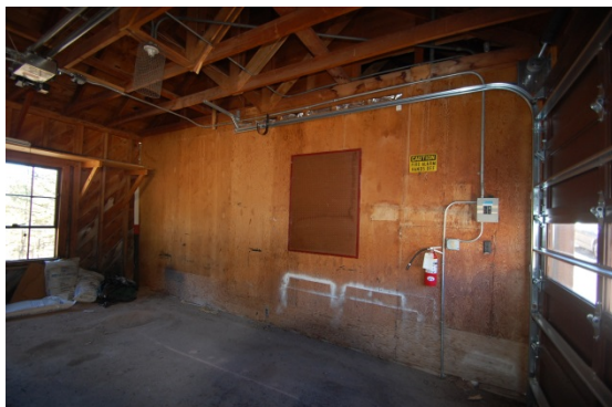
Figure 2-1. Garage 200 Looking at south wall. (SRJA 2014)
