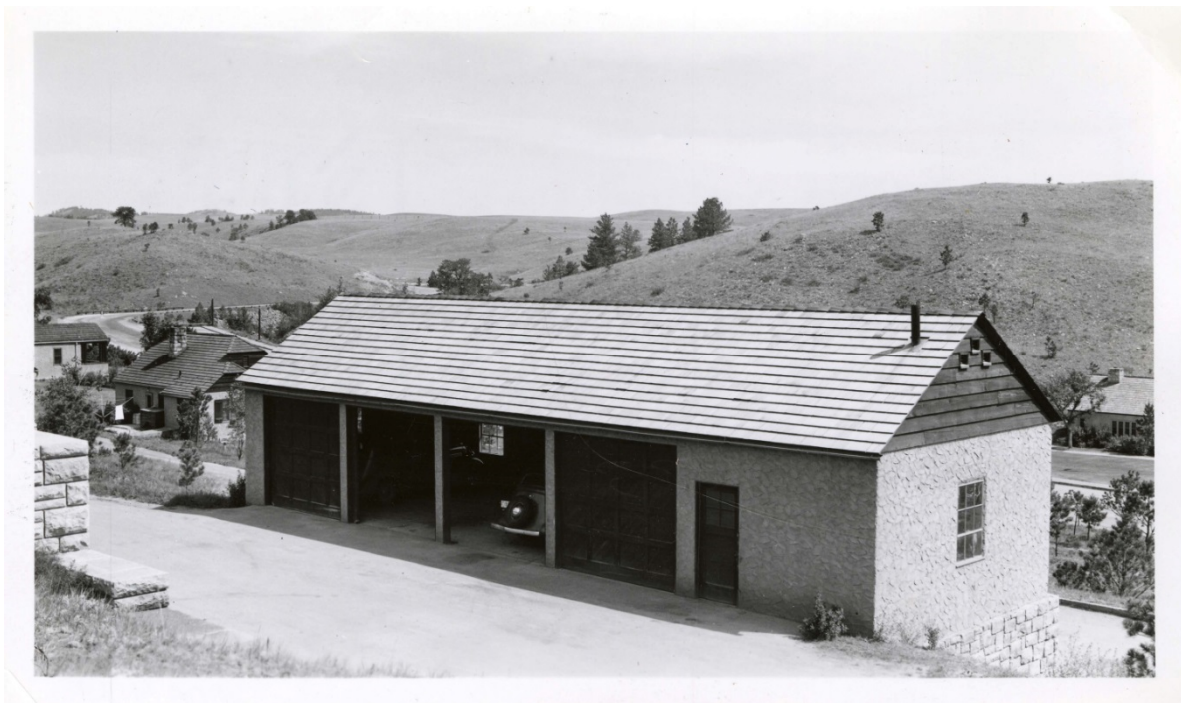
Figure 7. HS-11, ca.1938, looking northeast. (WICA 4129)
