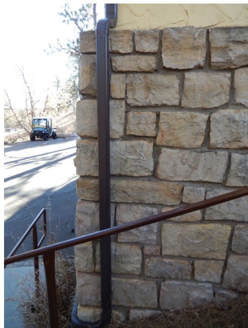
Figure X21. North Elevation detail at northeast corner. (SRJA 2014)
