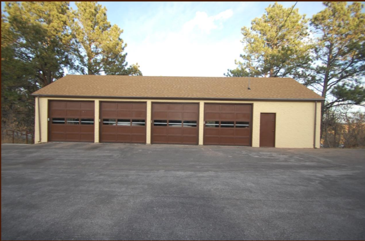
HS-11 West Elevation. (SRJA 2014)
