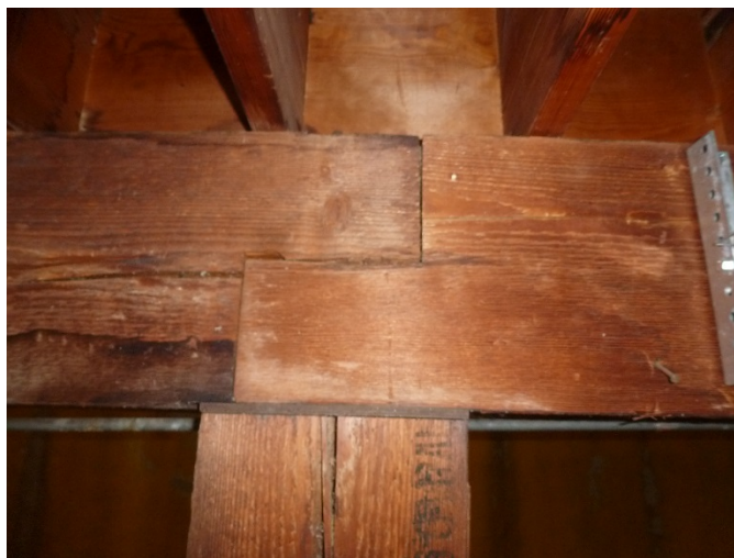
Figure S8. Girder splice on steel plate over post. (SEA 2015)
