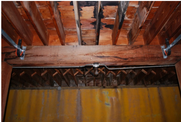
Figure 1-4. Garage 100 Looking west at second level floor framing, girder and west concrete foundation wall. (SRJA 2014)
