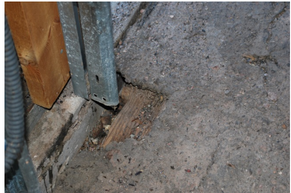
Figure 2-6. Garage 200 Detail at hole in floor near garage doors. (SRJA 2015)
