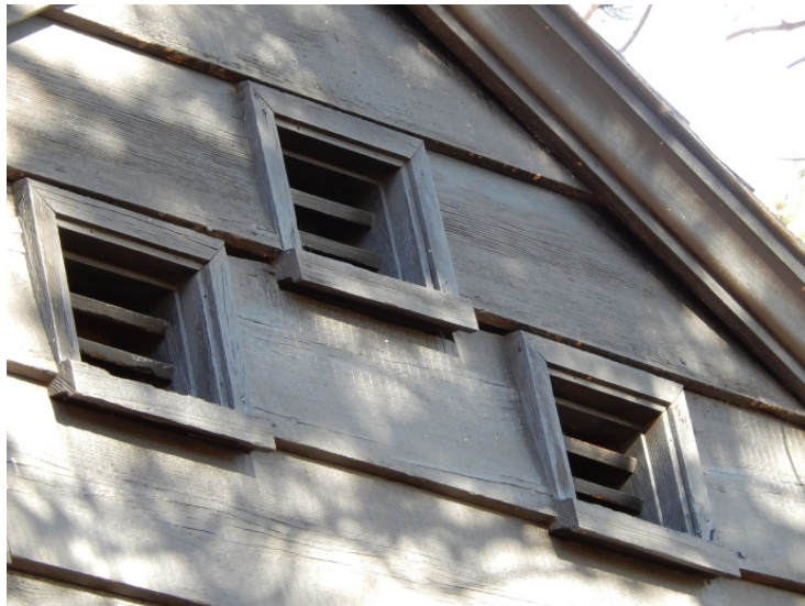
Figure X9. South Elevation detail of louvers. (SRJA 2015)
