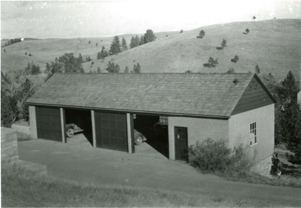
Figure 8. HS-11, ca.1940, looking northeast. (WICA 4557)
