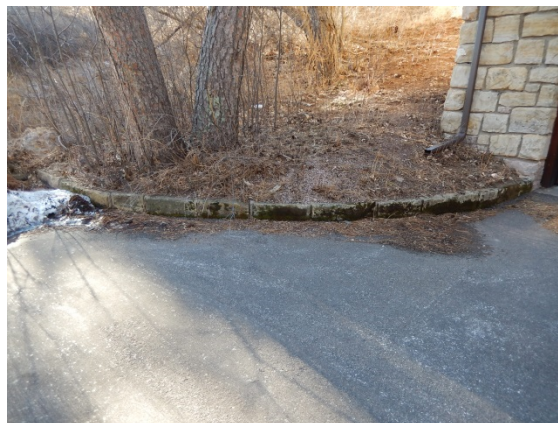
Figure X5. East Elevation detail at stone curbing. (SRJA 2015)
