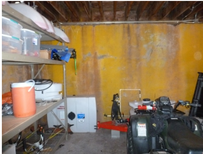
Figure S5. West foundation wall. (SEA 2015)
