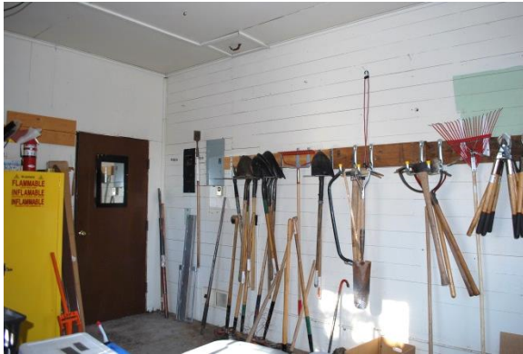
Figure 2-10. Room 201 Looking west and north. (SRJA 2014)
