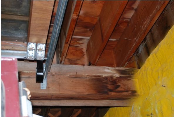
Figure 1-3. Garage 100 North end of girder pocketed into the north wall. (SRJA 2014)
