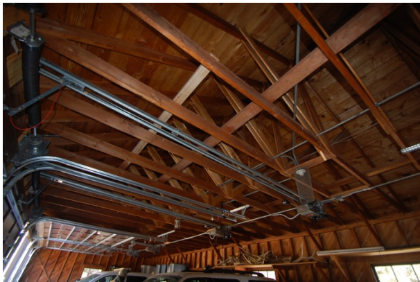
Figure 2-4. Garage 200 Looking north. (SRJA 2015)
