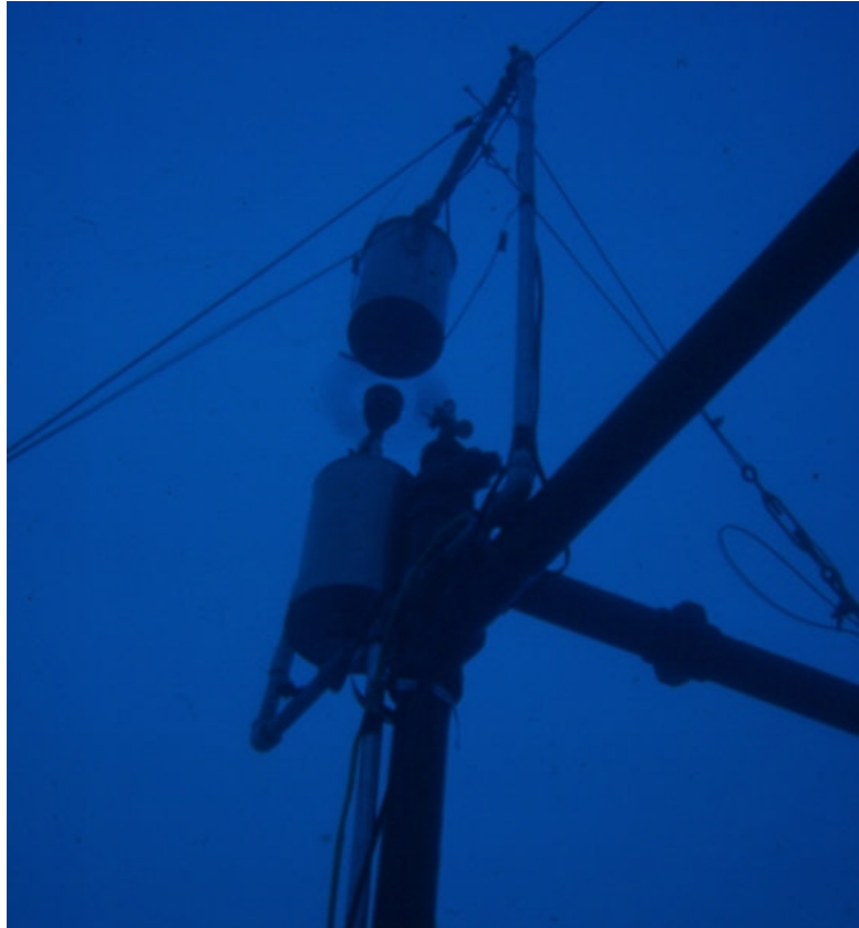
Shielded infrared heating tests, Old Mount Washington Observatory Tower, 1972-73. After D. E. Glidden
