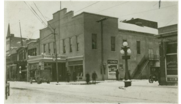
The Seneca Falls Garage on the corner of Fall and Mynderse Streets, ca. 1920.
