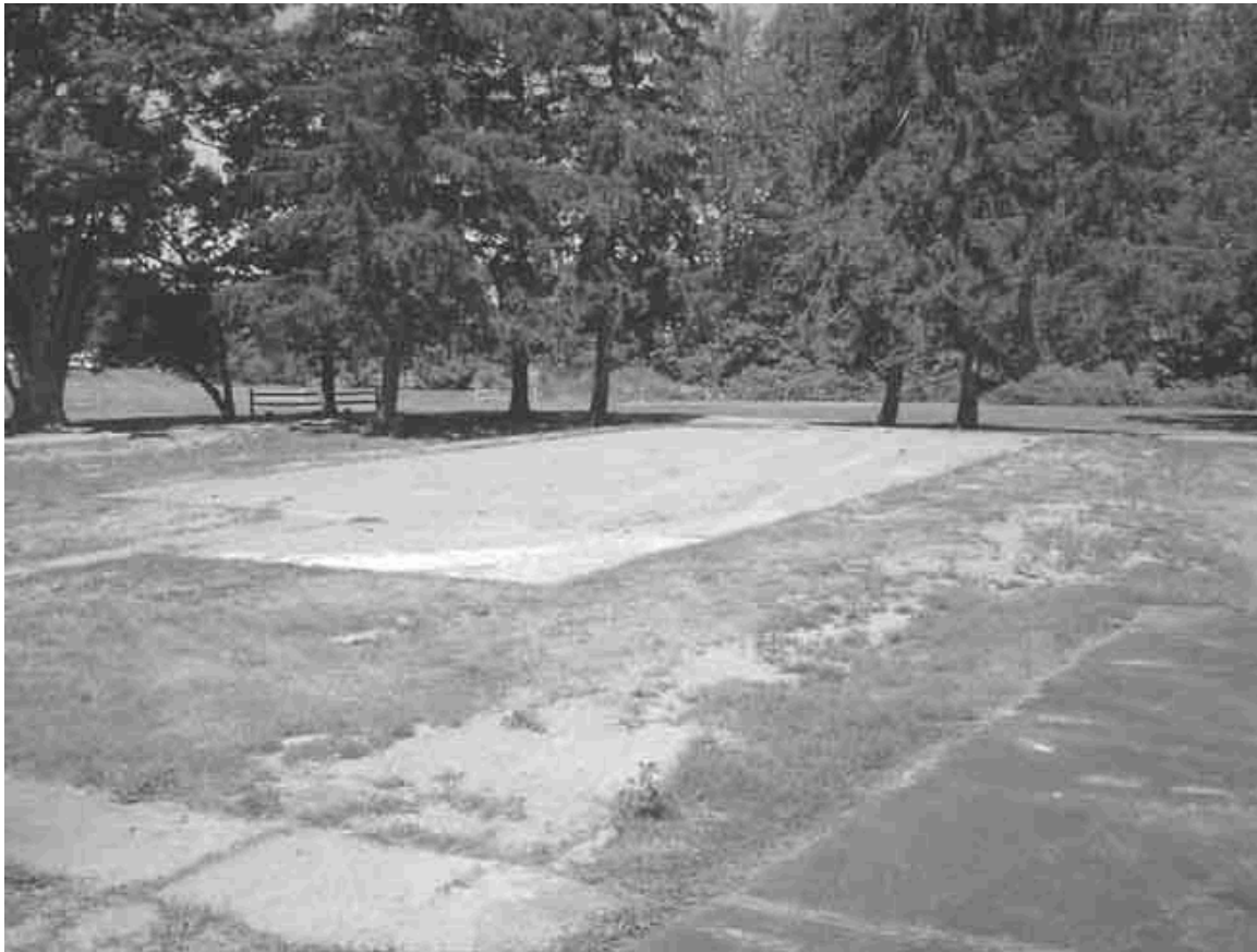
The swimming pool after the addition of fill material (SUNY ESF, 2001).
