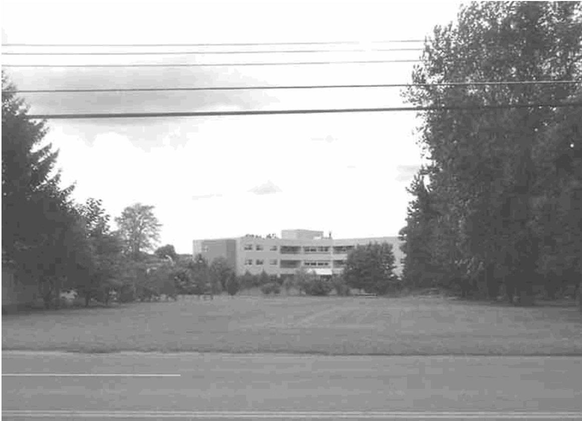
Health Center (lot 95) to the northwest of the Hunt House (SUNY ESF, 2001).
