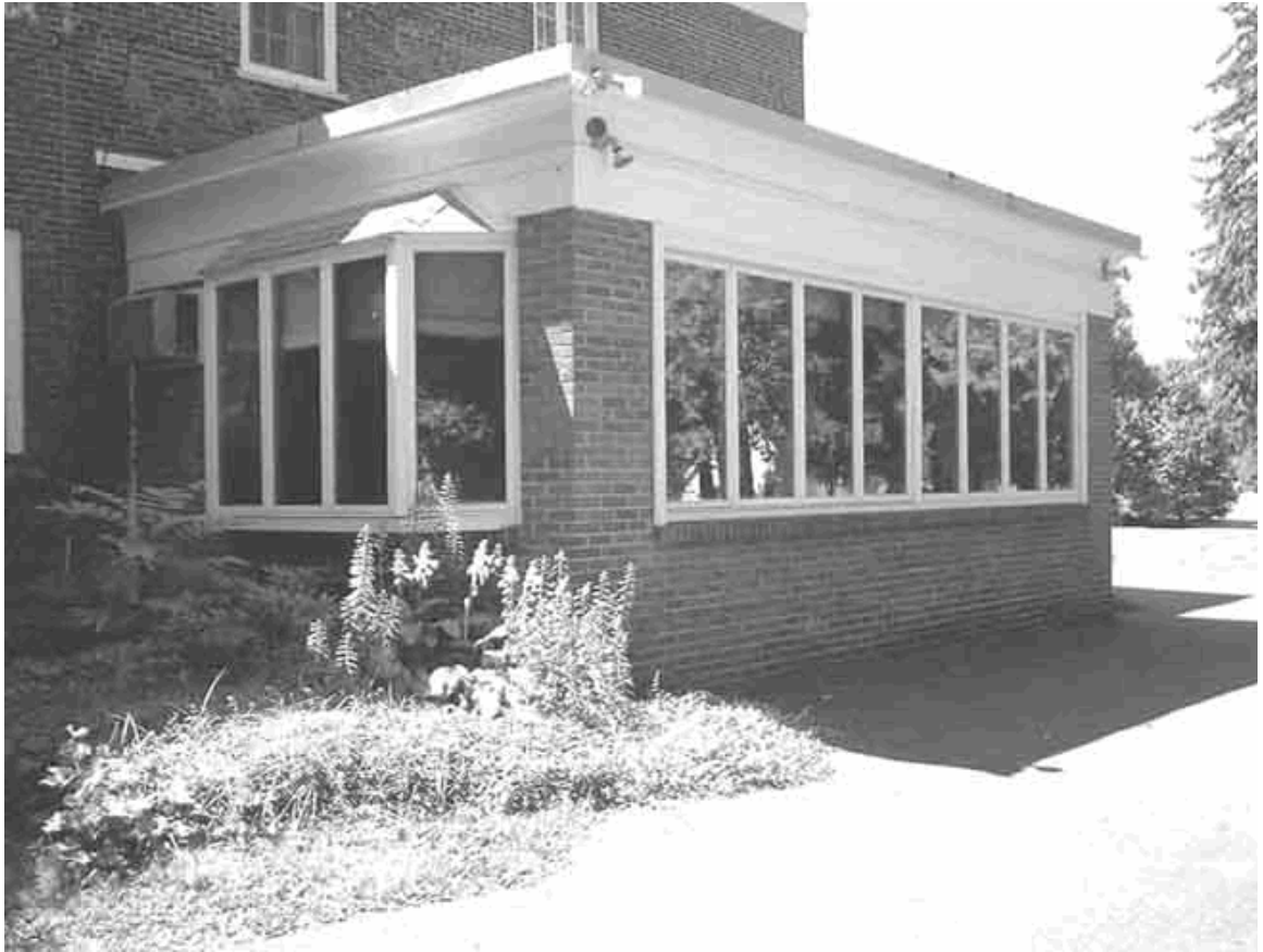
1960 addition to the north (rear) of the house (SUNY ESF, 2001).
