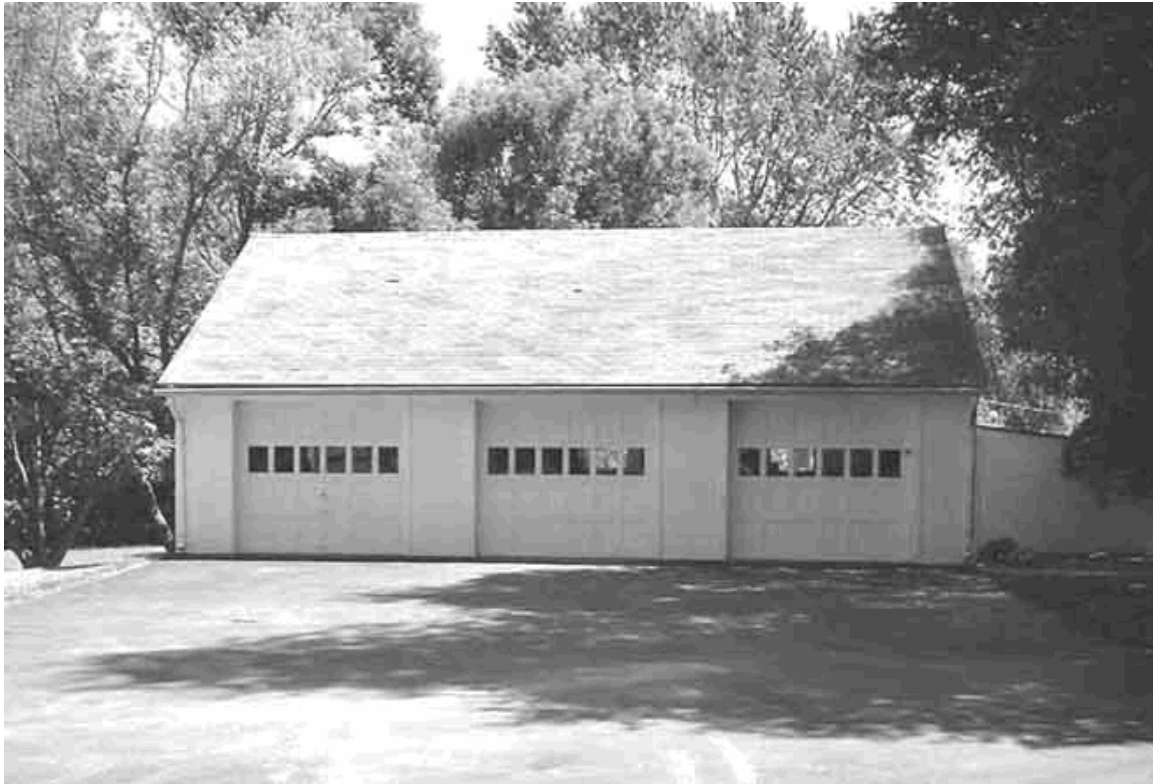
West side of the garage, constructed in 1954 (SUNY ESF, 2001).
