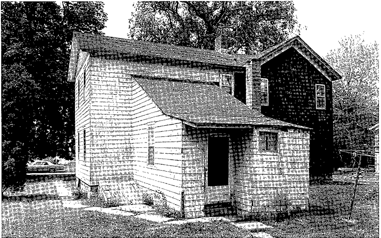
Figure 14. Stanton House: west and east elevations, July 19, 1968.
