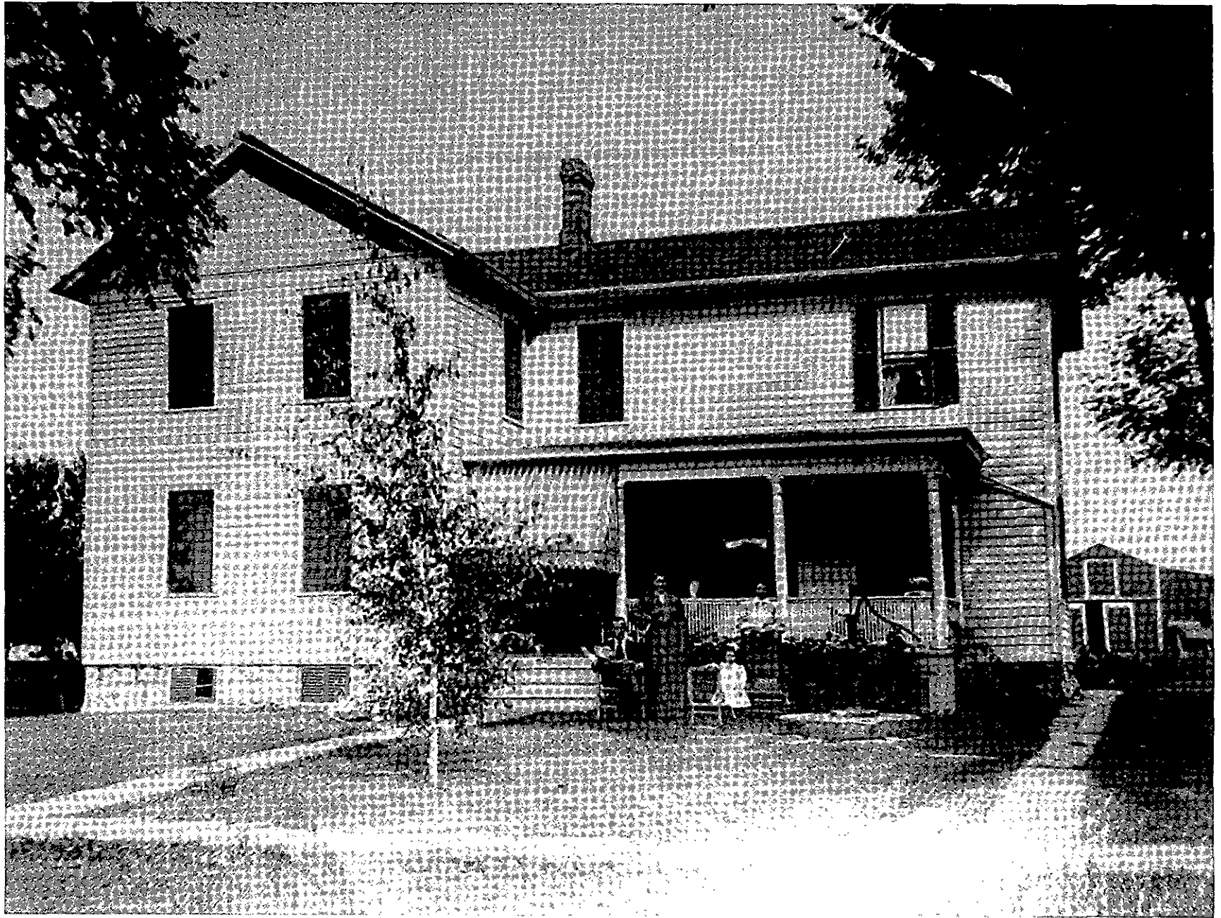
Figure 9. Stanton House: west elevation, circa 1904-05.
