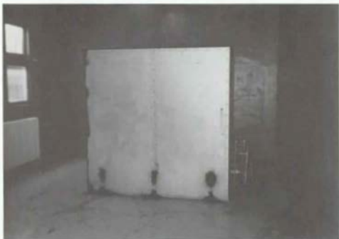
Fig. 50. Room 210 (Jail), Cell Block [1988].
