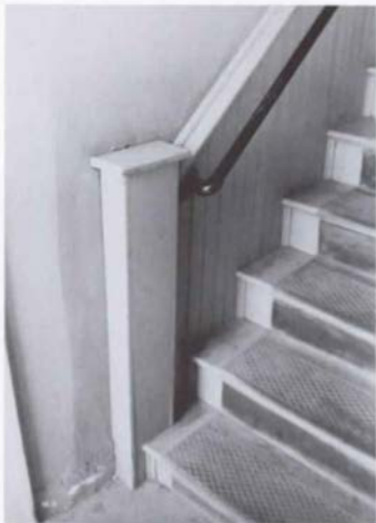
Fig. 24. Room 101 (Main Stairway) [1988].
