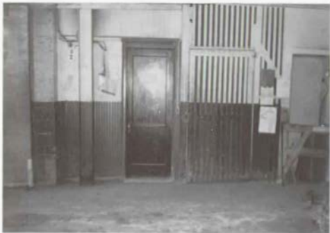
Fig. 35. Room 106 (Garage), Doorway to Toilet [1988].
