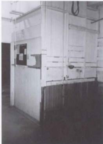
Fig. 37. Room 109 (Water Department), Northwest Corner [1988].
