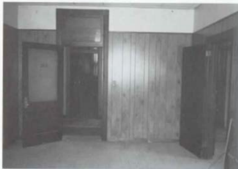
Fig. 53. Room 216 (Investigator's Office), West Wall [1988].
