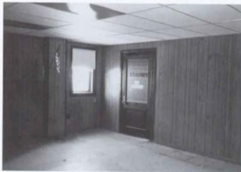
Fig. 42. Room 203 (Police Locker Room), Southeast Corner [1988].
