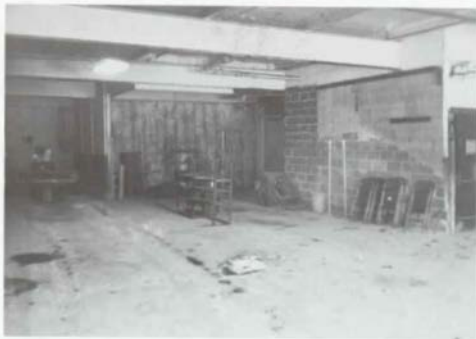
Fig. 33. Room 106 (Garage), Looking Southwest [1988].
