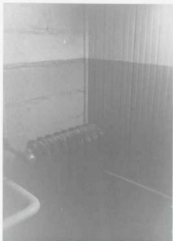
Fig. 36. Room 108 (Toilet), Northeast Corner [1988].
