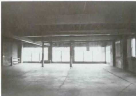
Fig. 57. Third Floor, Looking South [1988].
