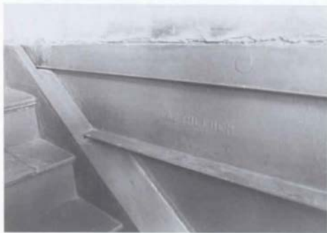
Fig. 41. Room 201 (Main Stairway) [1988].
