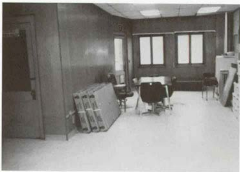
Fig. 25. Room 102 (Village Office), Looking South [1988].
