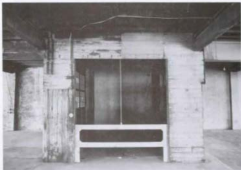
Fig. 58. Third-Floor Elevator Enclosure [1988].
