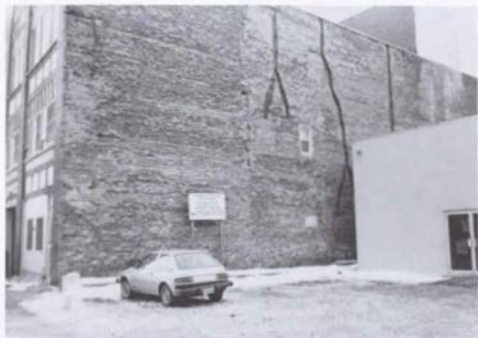
Fig. 17. Exterior East Wall [1988].
