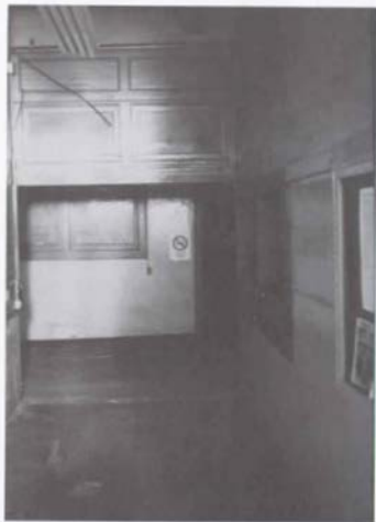
Fig. 43. Room 204 (Dispatcher Room), Looking North [1988].
