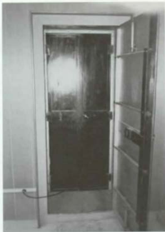
Fig. 27. Room 102 (Village Office), Doorway to Vault [1988].
