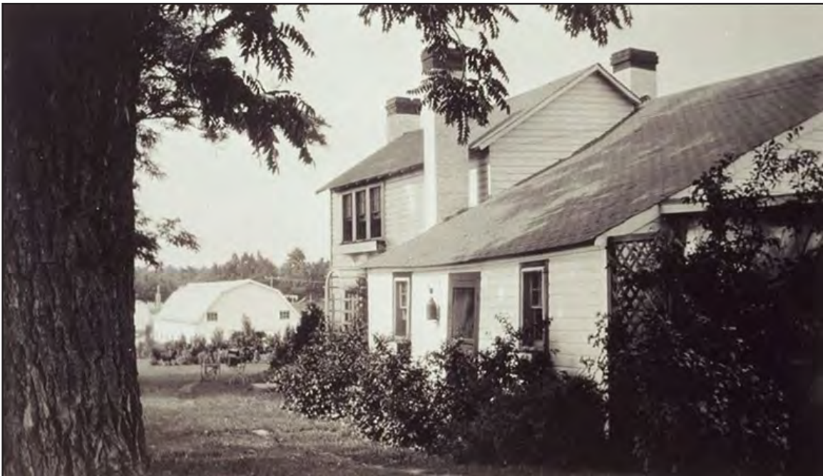
FIGURE 13: View of the Main House ca. 1935 with the Stone Kitchen Addition (Harvard University, Schlesinger Library)
