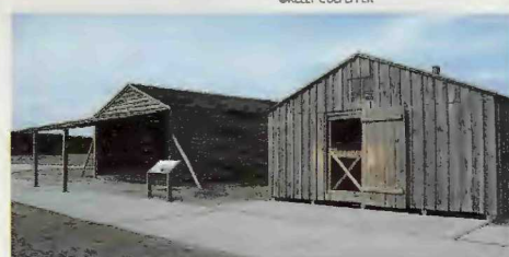
Reconstructed 1903 Hangar and Quarters/Workshop
