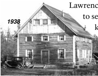
photo: G. Bleakley collection
