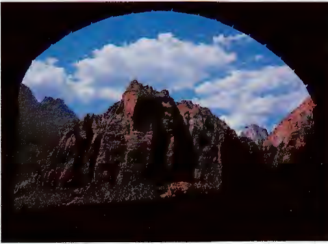
View out long tunnel
