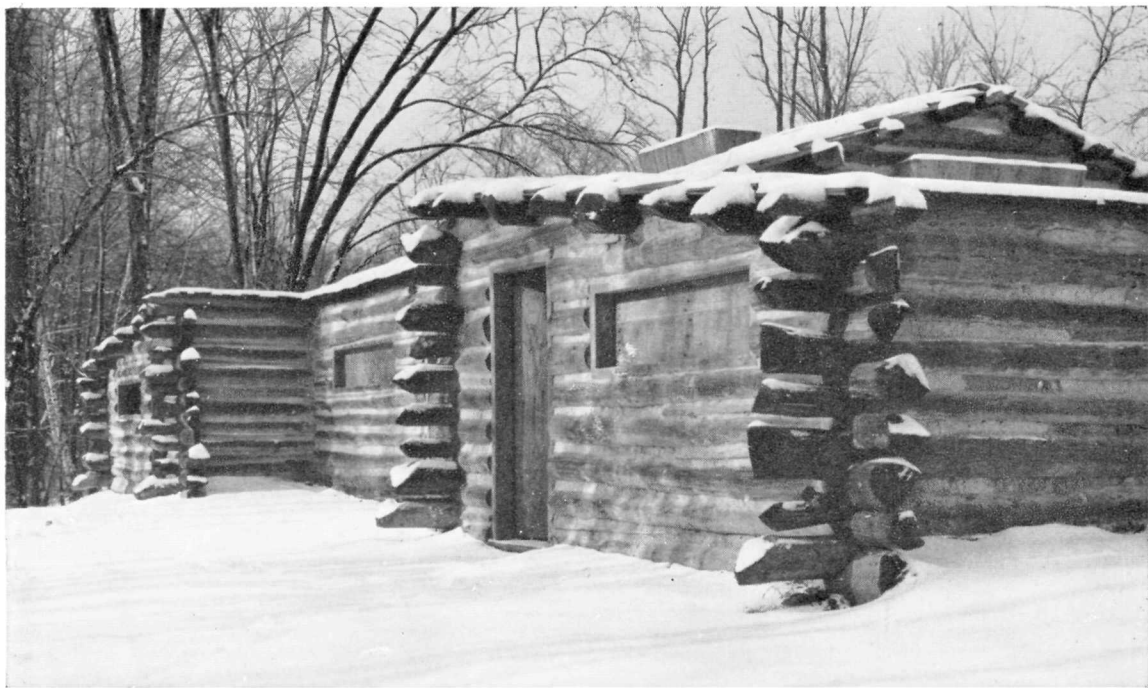
Reconstruction of Continental Army hospital hut built in the winter of 1779 in what now is Morristown National Historical Park, N. J. Fires on the earthen floor provided the only heat. Smoke escaped through the wooden vents in the roof.
