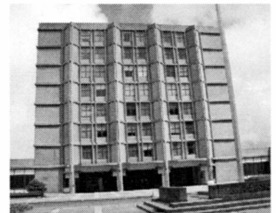
Letterman Army Medical Center, to be demolished.
